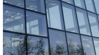
SSG CURTAIN WALL TGP Steelbuilt Curtainwall Infinity SSG System
