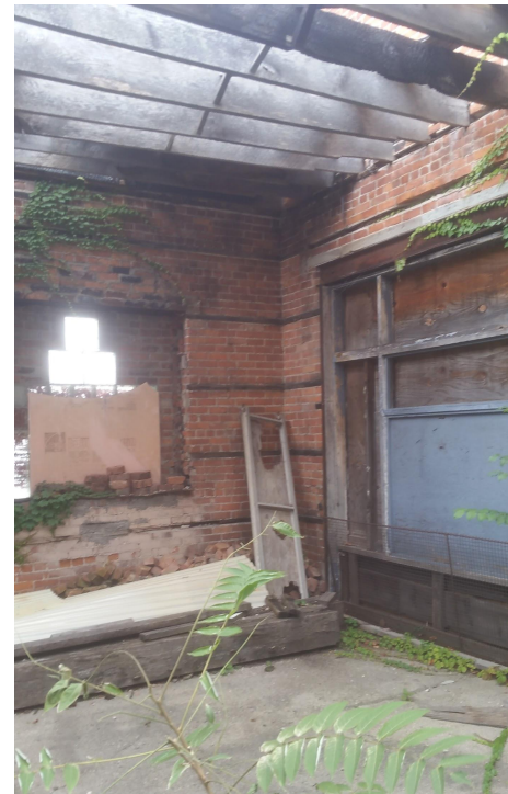
INTERIOR NORTH-EAST CORNER
