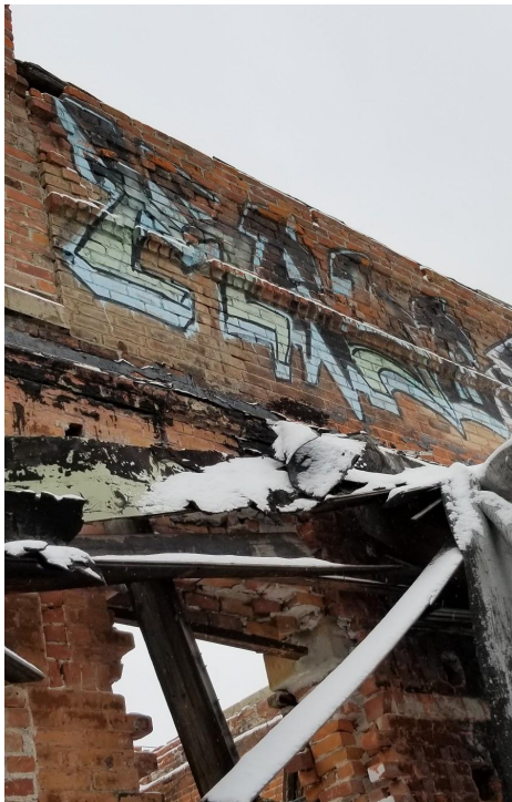
INTERIOR LOOKING EAST
