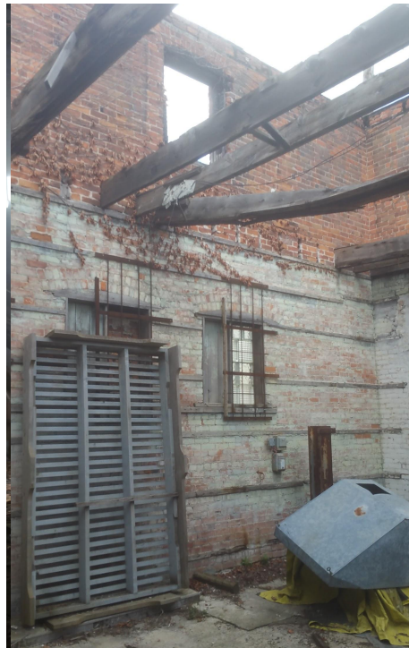
INTERIOR NORTH-WEST CORNER
