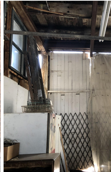
1 STORY SOUTH WINDOWS
