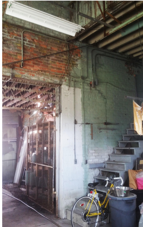
INTERIOR LOOKING NORTH
