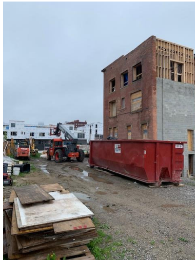
Side Yard View
