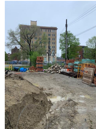
Building Site – Looking West
