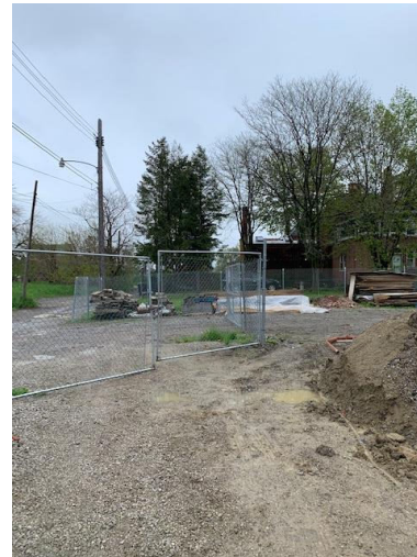
Building Site – Looking East
