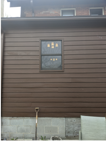
Window to be replaced:
