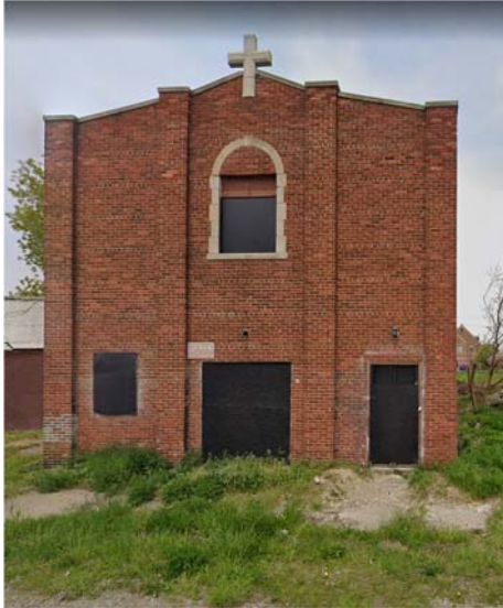
Existing Condition (South Elevation)
