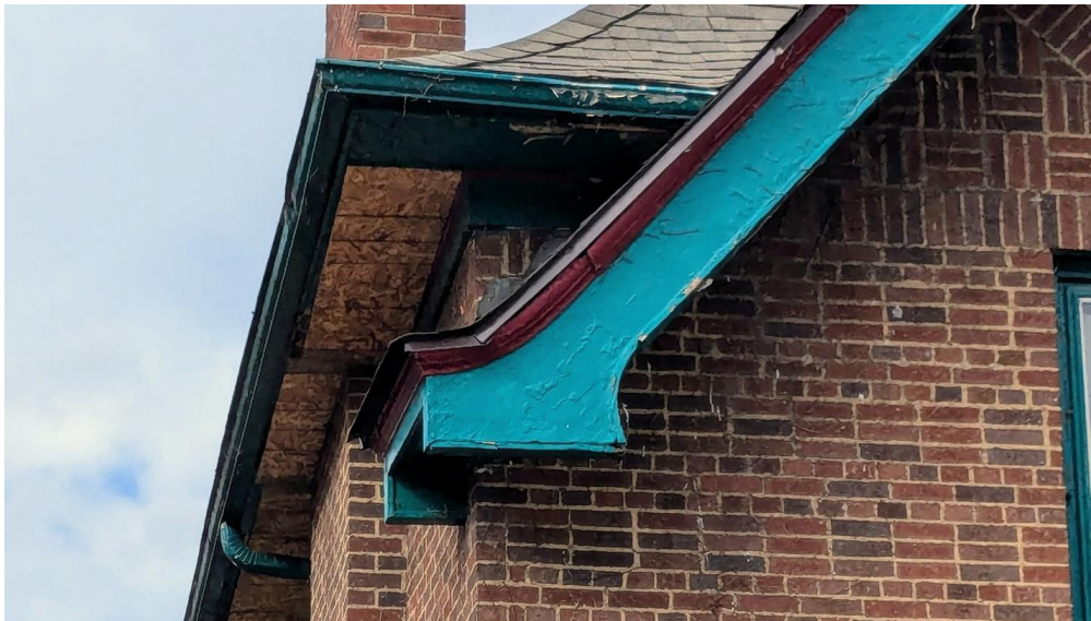
Area of lost soffit material. February 2025 photo by staff.
