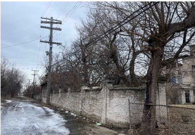
Site Photo 1, by Staff February 28, 2025: Arden Park HD, Brush Street between Belmont and East Boston Boulevard (facing east) showing alley and overhead powerline conditions. The branches and trunks that are within 15' of the overhead lines or poles are subject to "enhanced" maintenance according to this proposal. See figure 1.
