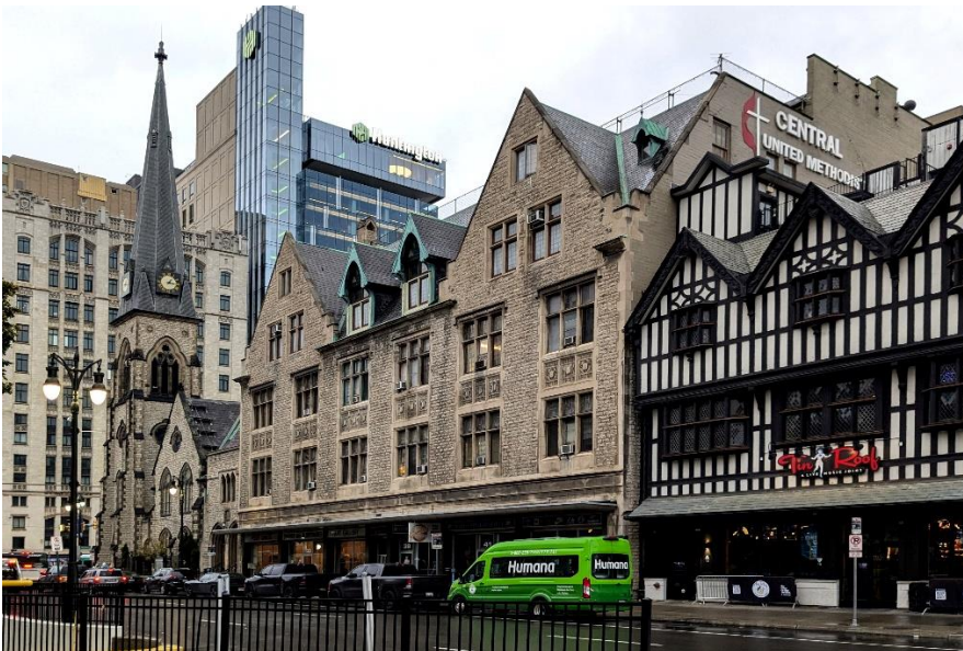
Central United Methodist Church with 1914–1916 addition (31 E. Adams) in foreground, center of image. November 2024 photo by staff.
