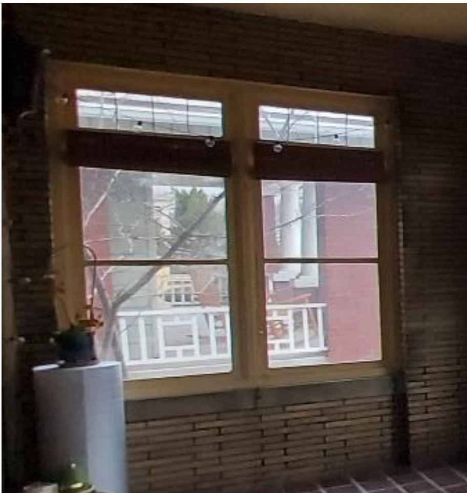
Window type that is present at the porch, front façade, first story. This window was installed ca. 1984. The window type is a wood 1/1 unit with what appears to be a fixed transom with metal casing
