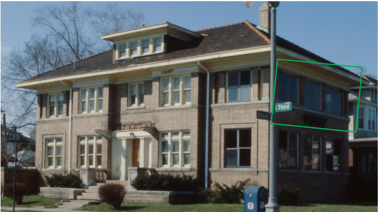
801 Edison, photo taken in 1980. See the side porch wing. The windows at the porch outlined in green are jalousie windows. All other windows at the porch appear to be 1/1 storm windows
