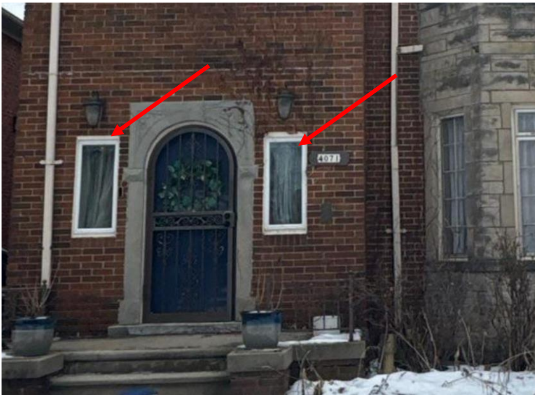
Front façade vinyl windows added ca. 2013. Proposed for replacement with aluminum-clad wood units, indicated by arrows. Photo by applicant
