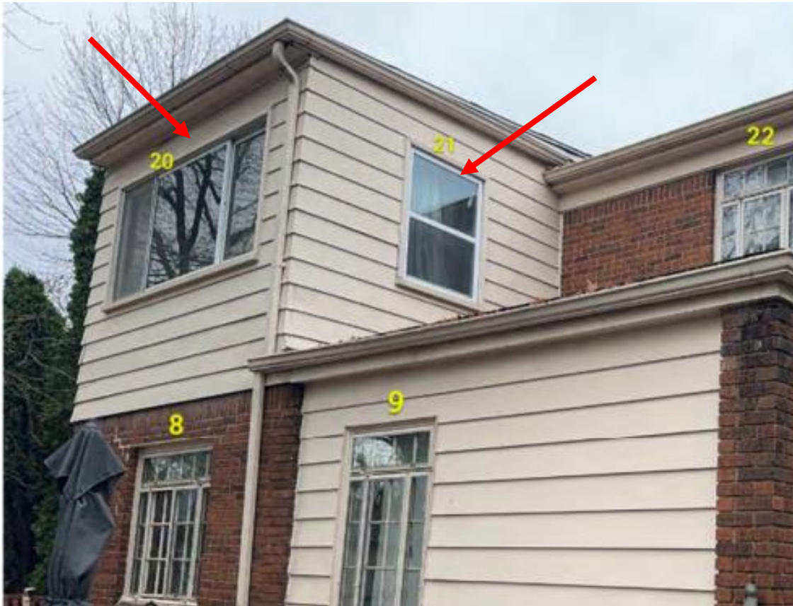
Rear second story porch, erected in 1967. Vinyl windows proposed for replacement with aluminum-clad wood units, indicated by arrows. Photo by applicant
