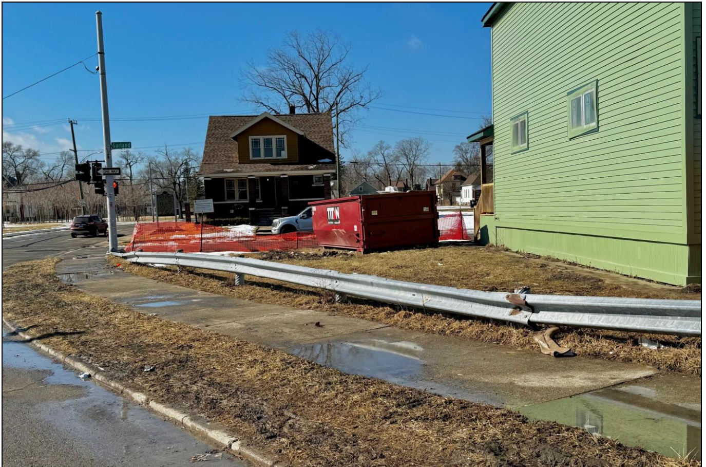
Looking west from Charlevoix, which is the direction of automobile traffic, this view captures the façade of the Ossian Sweet house directly behind the public right-of-way. Staff photo, February 2025.
