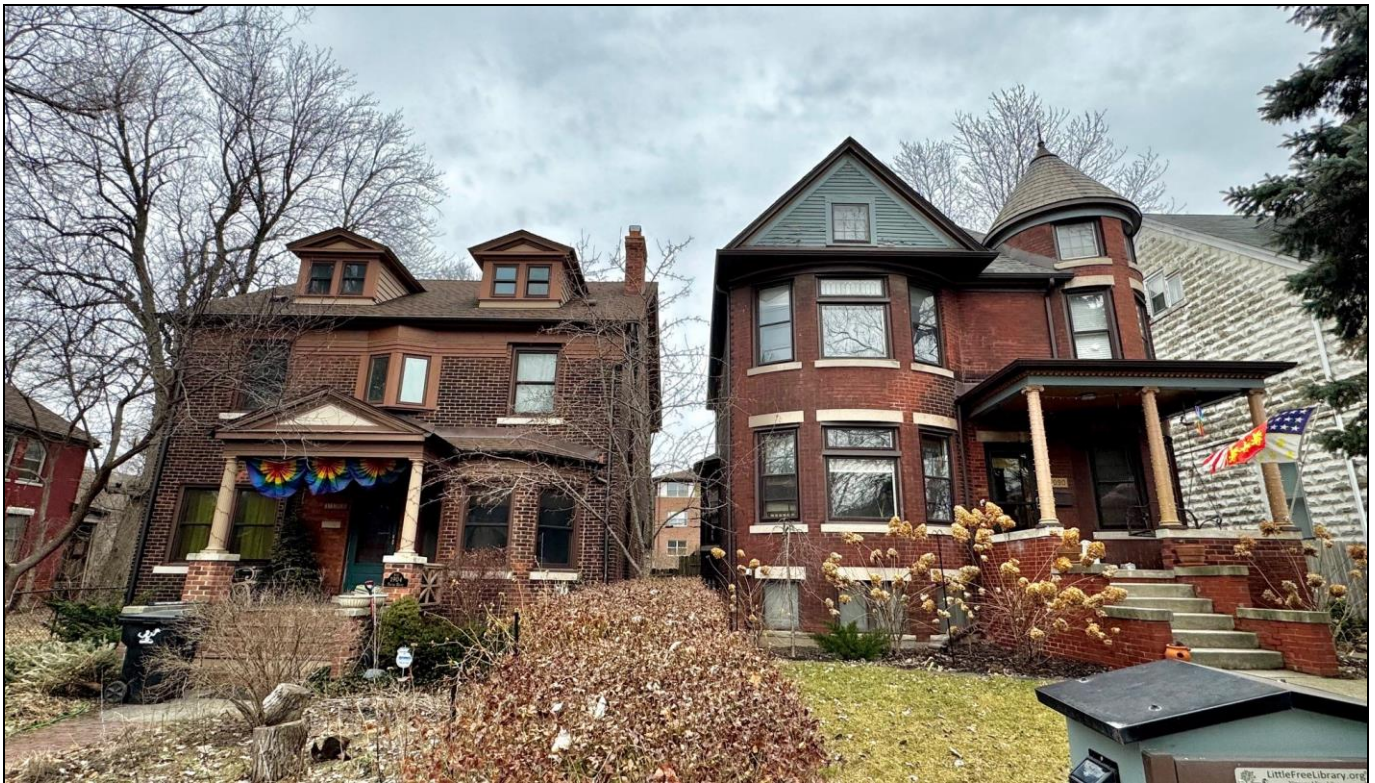
This view on Vinewood, looking directly east, documents the proximity of the adjacent house to the north. Staff photo, February 28, 2025. This photo was taken at the sidewalk, which is approximately three feet higher than the roadway. The lawns on this side of the street also rise from the sidewalk, the raised basement at 1090 Vinewood further increases the distance of the roof from the sidewalk, which will help obscure the proposed dormer from the street.
