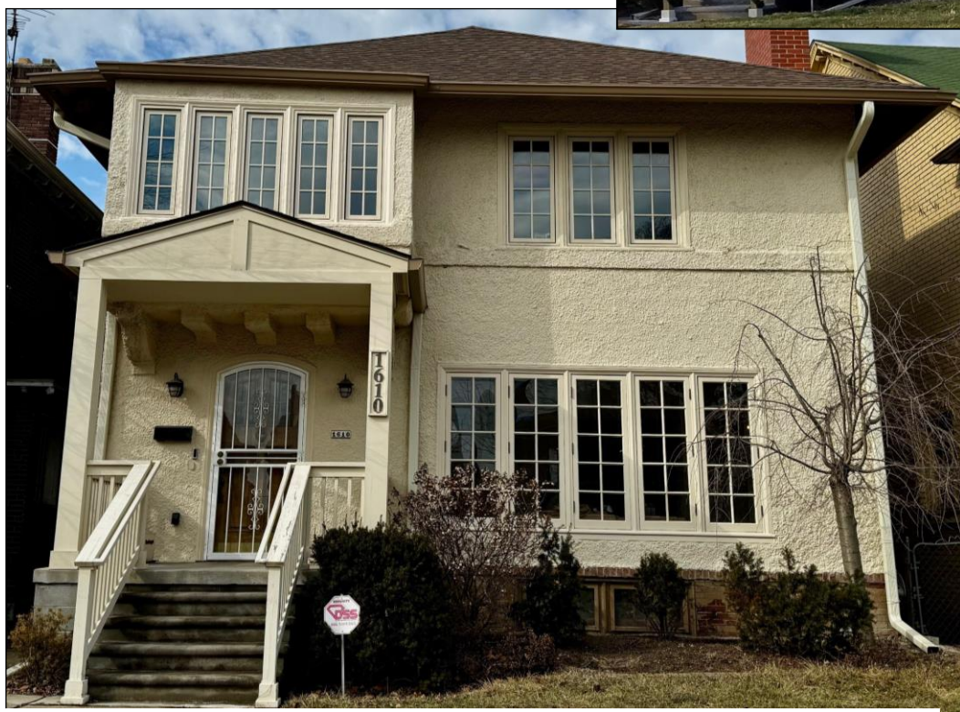
Above: Current conditions - The repair and finish work to the stucco at the bottom of the box bay, as well as the area above the grouped window shows minimal, if any, evidence of the former awnings.
