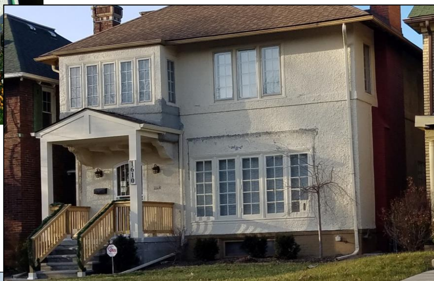
Above: This 2019 photo shows the lower wall of the upper porch has been rebuilt, and evidence of the awning at the first floor grouped window opening is still visible. Staff photo, January 6, 2019.
