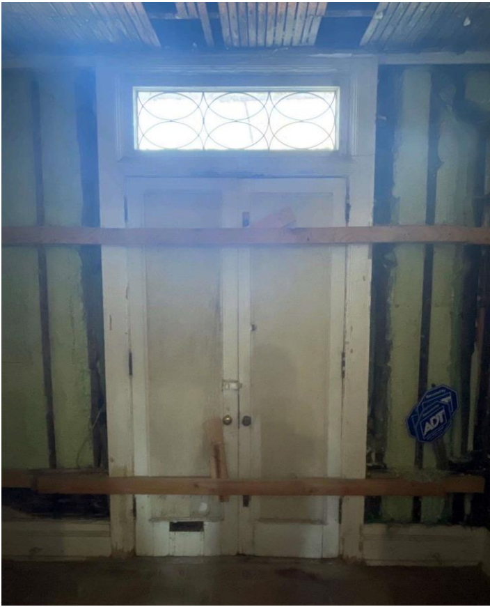
Applicant photographs. The interior framing understandably exhibits less weathering than the exterior, and only requires spot repairs and repainting, as well as the new glass for the doors.
