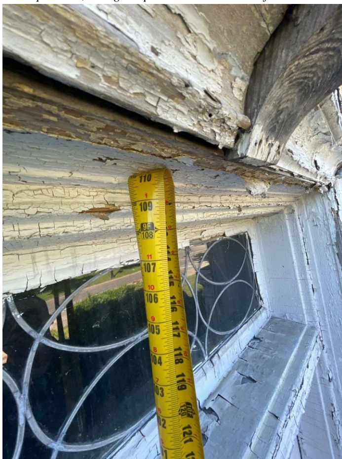
Applicant photographs. The entire entry surround requires repair and repainting, and that missing elements be fabricated and installed. For this application's scope of work, the transom window (glass and lead cames) and French doors are intact and repairable; new glass panels can be ordered for the doors.
