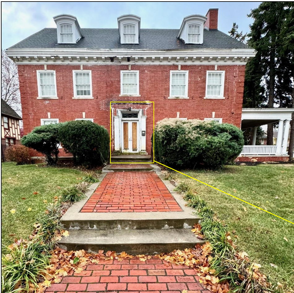
Façade facing Chicago Boulevard.
