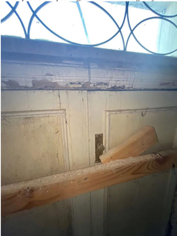
Applicant photographs. The interior framing understandably exhibits less weathering than the exterior, and only requires spot repairs and repainting, as well as the new glass for the doors.
