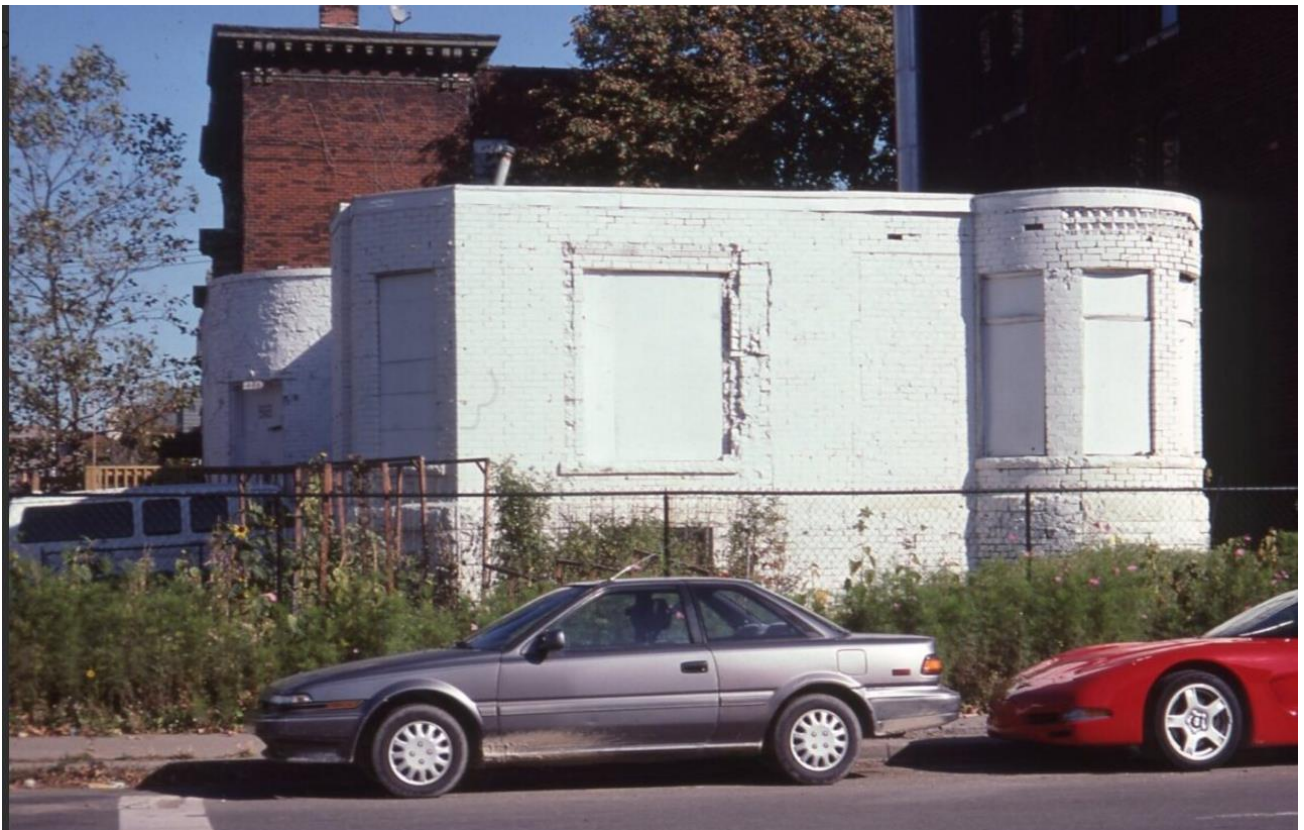
Designation slide showing appearance in 2000. HDAB
