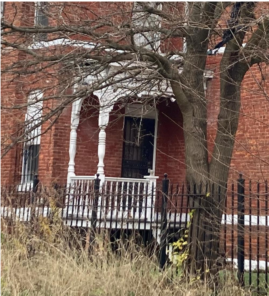
East side porch proposed for demolition, HDC staff 11/25/2024
