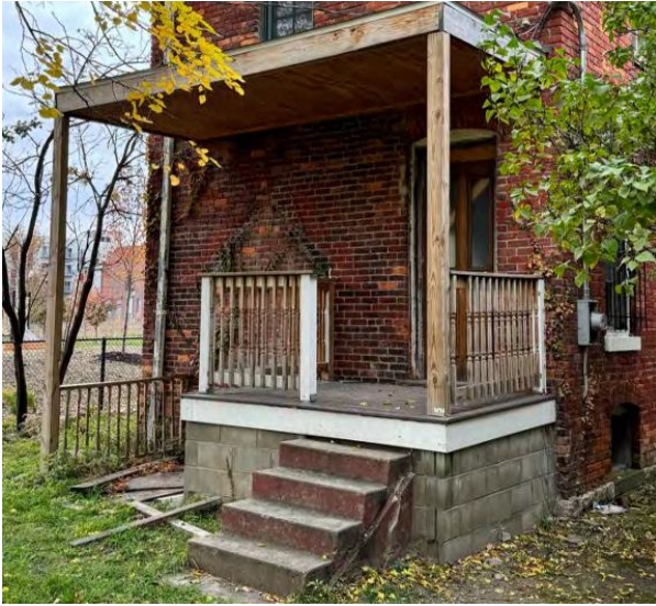
Current rear porch proposed for removal.
