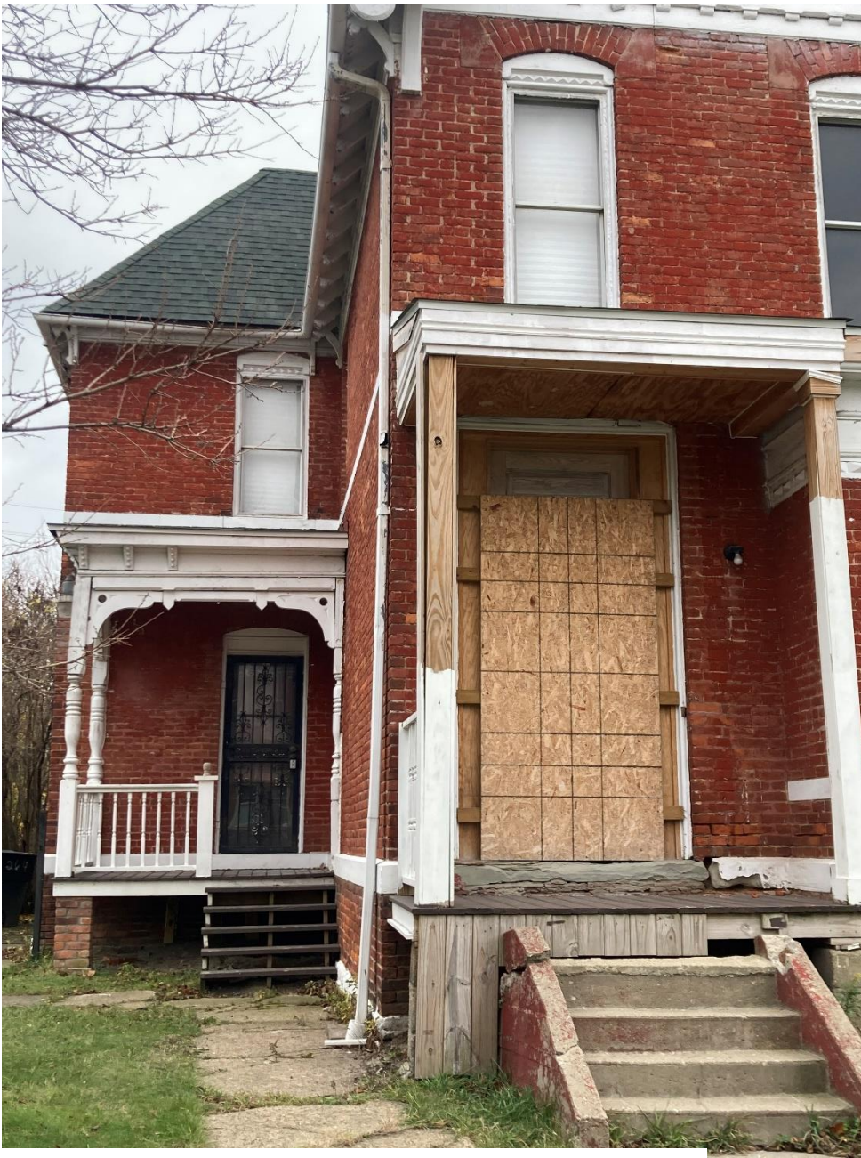
East side porch proposed for demolition, HDC staff 11/25/2024
