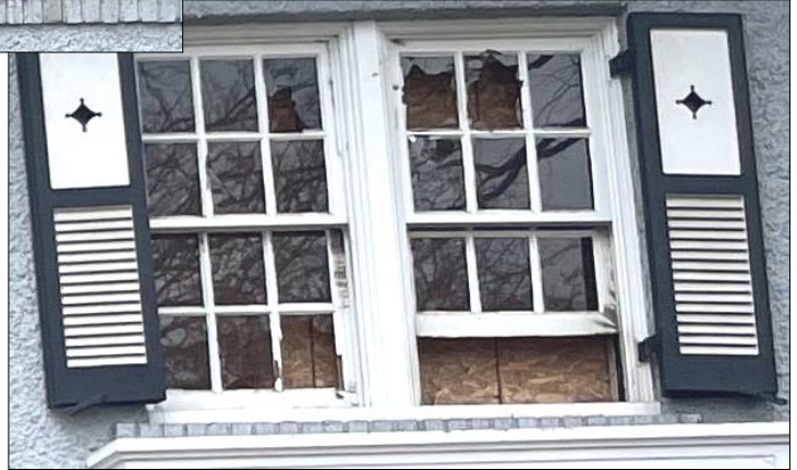
HDC staff photos taken on February 13, 2024 shortly after the fire. These photos show smoke on all the window frames, as well as several glass panels broken at the second story.
