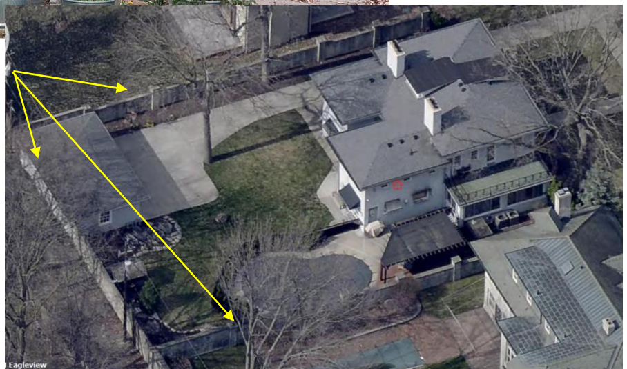
Right: Aerial view of the property. Concrete walls are visible from this viewpoint.
