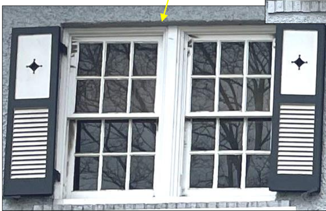
HDC staff photos taken on February 13, 2024 shortly after the fire. These photos show smoke on all the window frames, as well as several glass panels broken at the second story.
