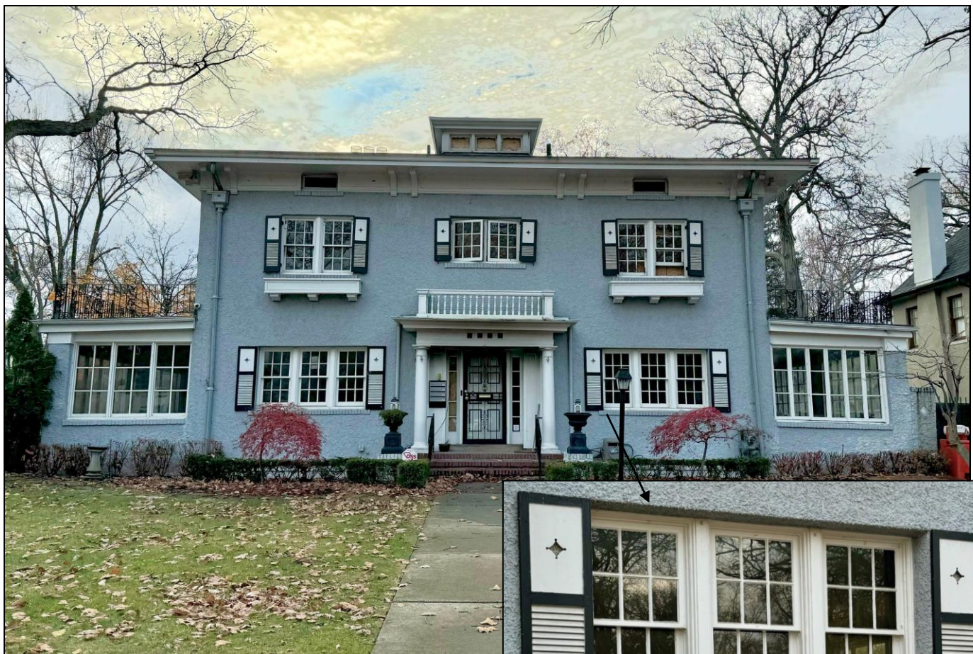
Facade of house. Staff photos, November 26, 2024.
