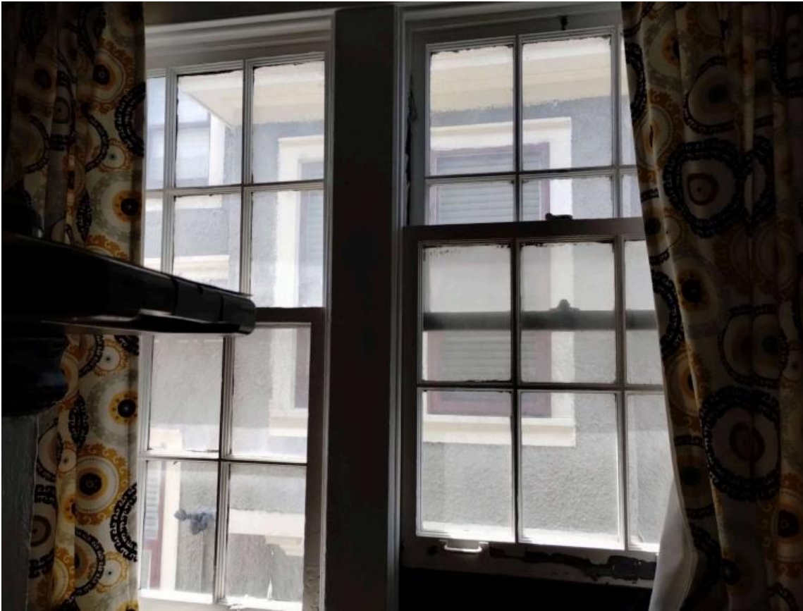
Windows proposed for replacement, interior. Photo provided by applicant
