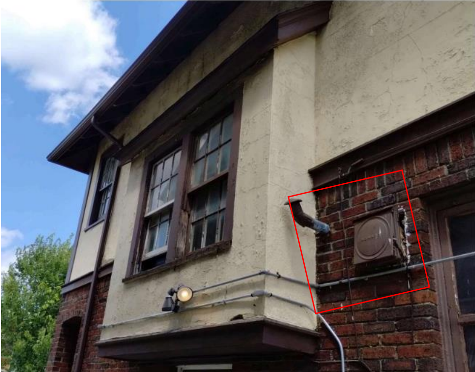
Vent proposed for removal (outlined in red). Photo provided by applicant
