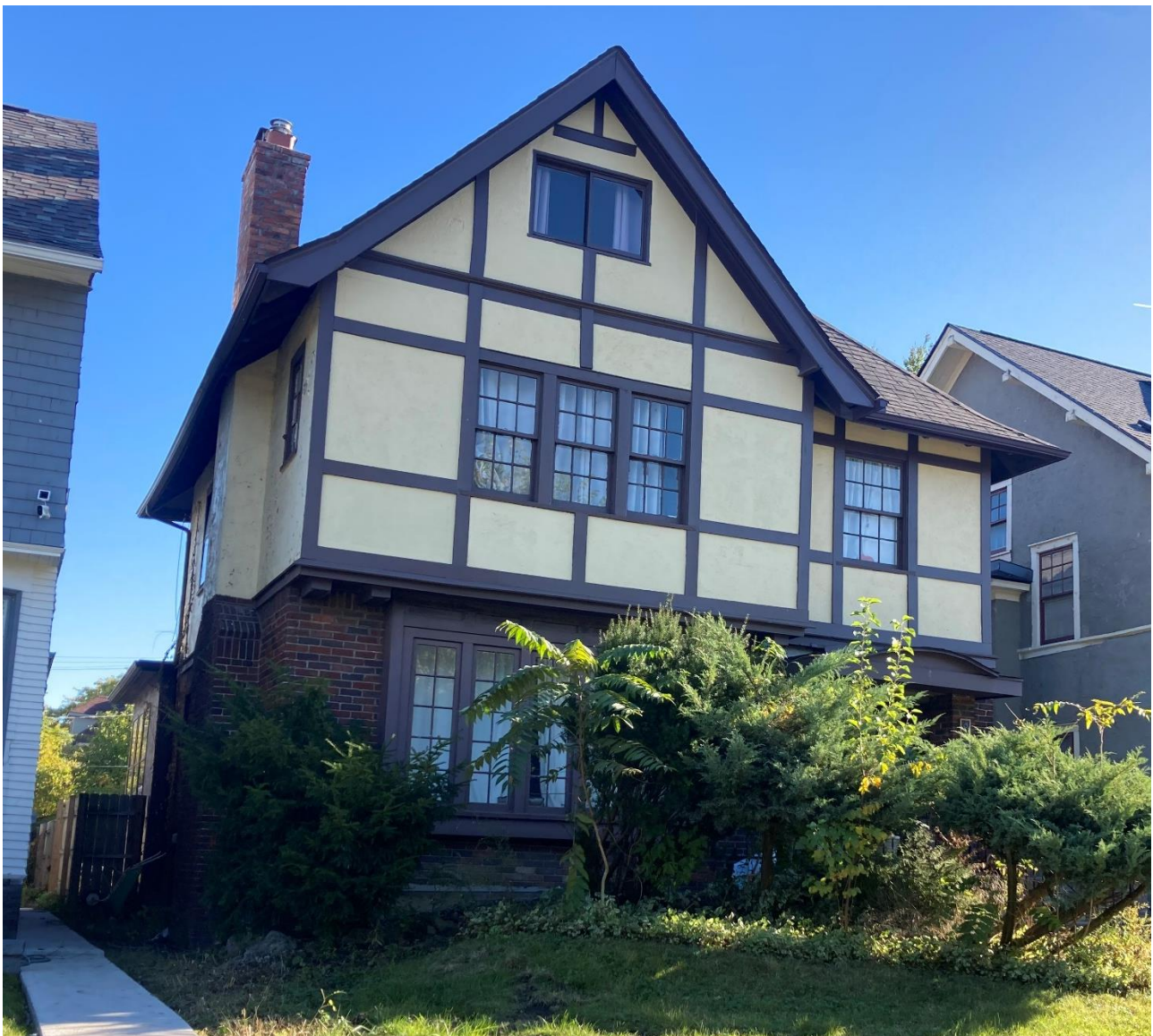
Current condition, staff photo taken on 10/16/2024
