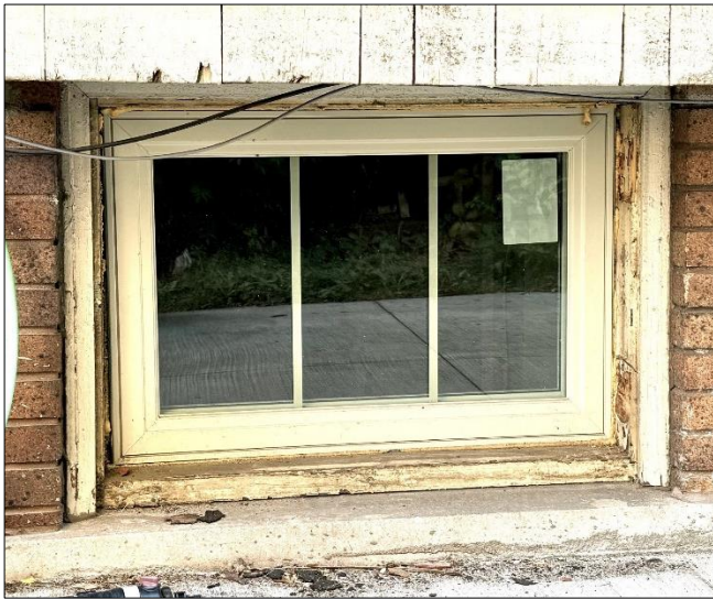
Basement window openings.
