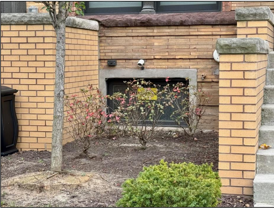
Location of proposed egress window/window well. Staff photo, November 1, 2024.
