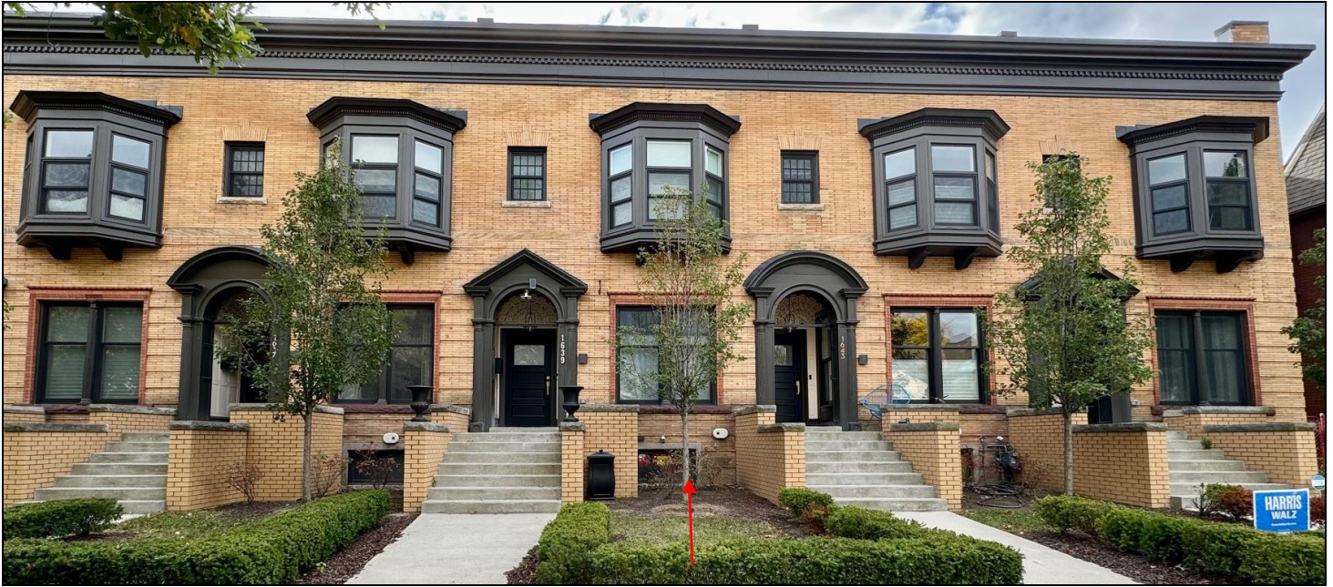
Existing conditions. Staff photo, November 1, 2024. Location of window.
