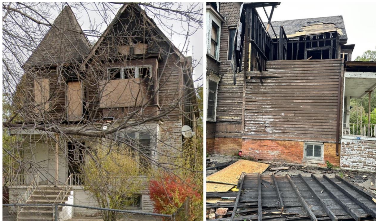
Left: November 2020 photo from Google Street View. Right: Image from 2023 application documents, view from the north. Note that the pyramidal roof tower is missing; red arrow is added by staff to indicate former tower location.
