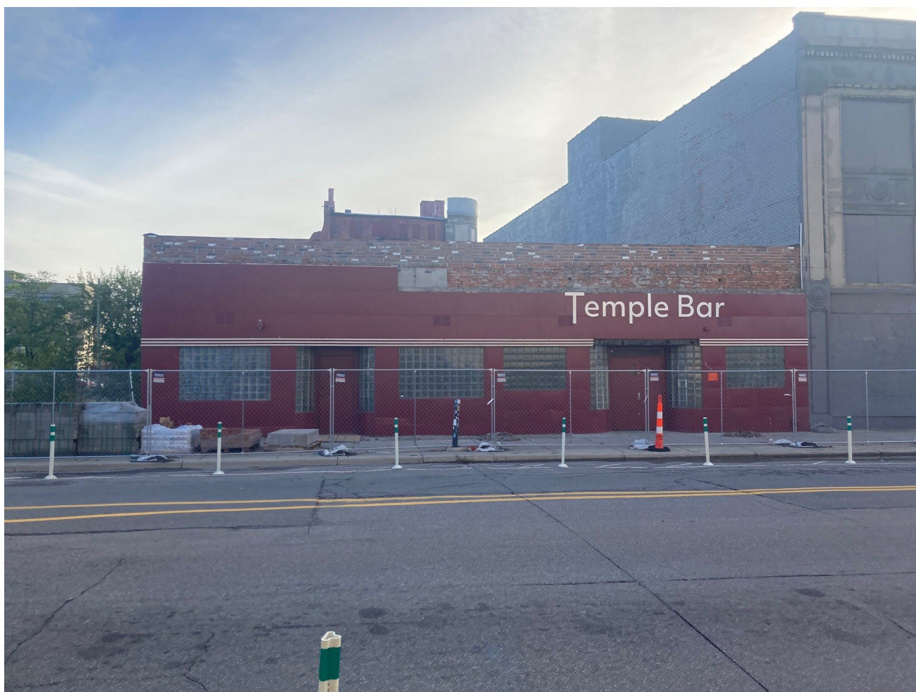
Figure 1: Current view of 2906 Cass, looking east.
