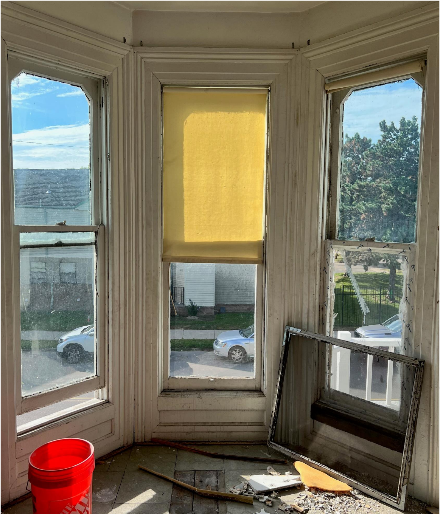
First floor bay windows – interior – historic windows
