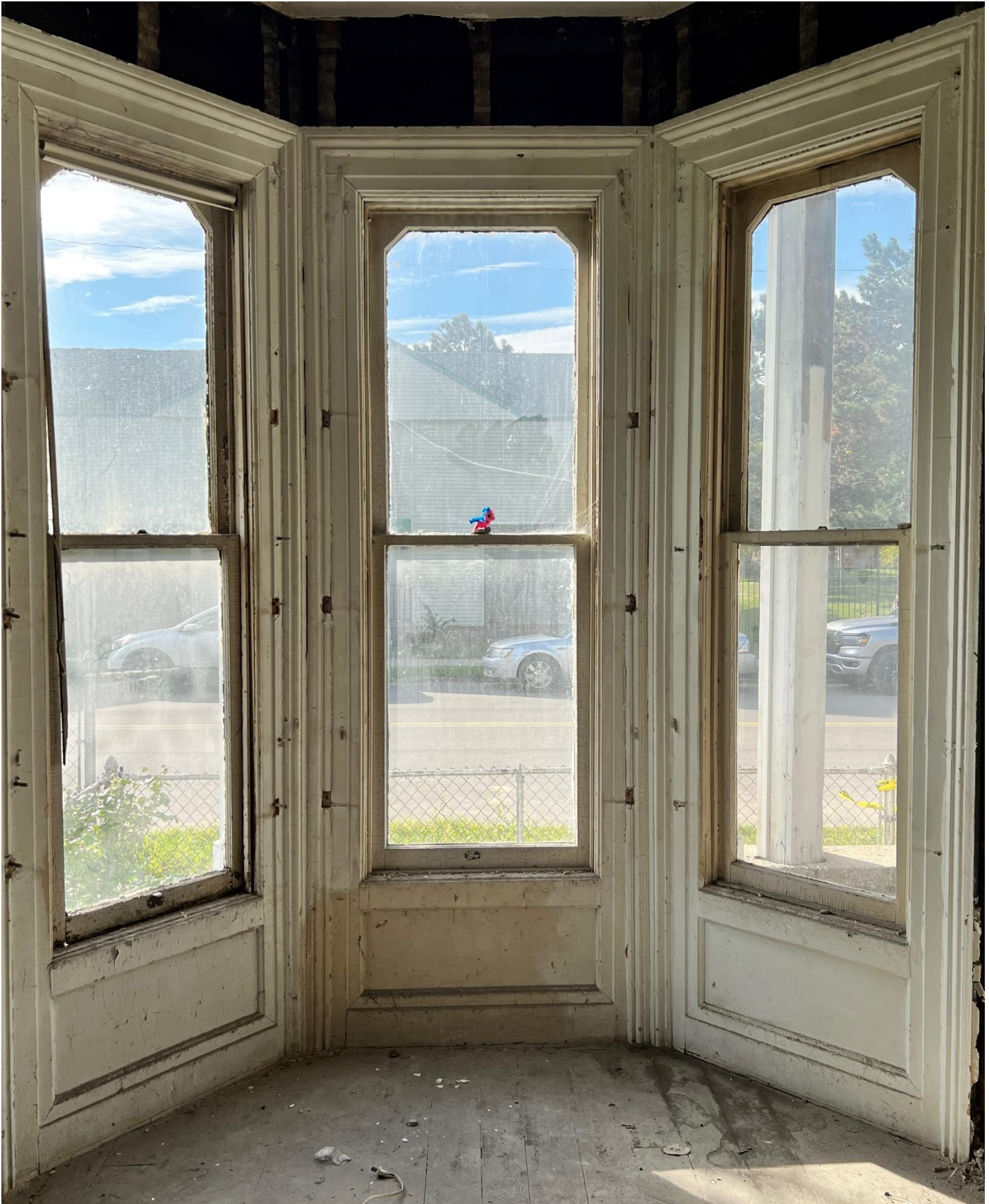
First floor bay windows – interior – historic windows
