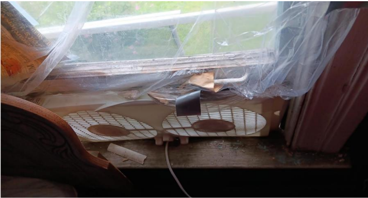
WINDOW D – Covered with plastic Photo by applicant
