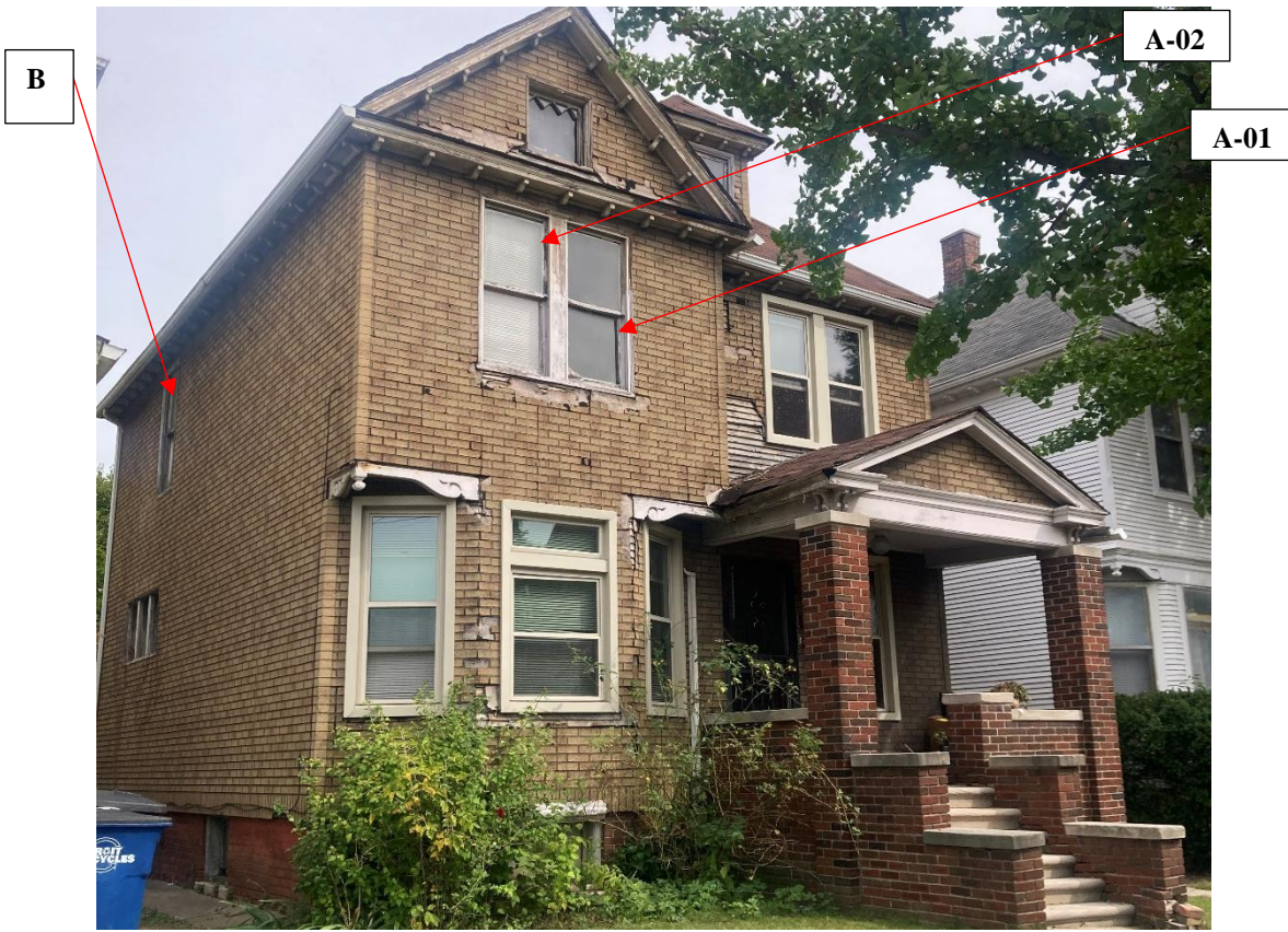
Staff photo taken on 10/3/2024. Front and side wall
