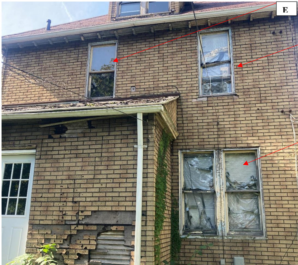
Rear wall, photo taken by HDC staff on 10/3/2024
