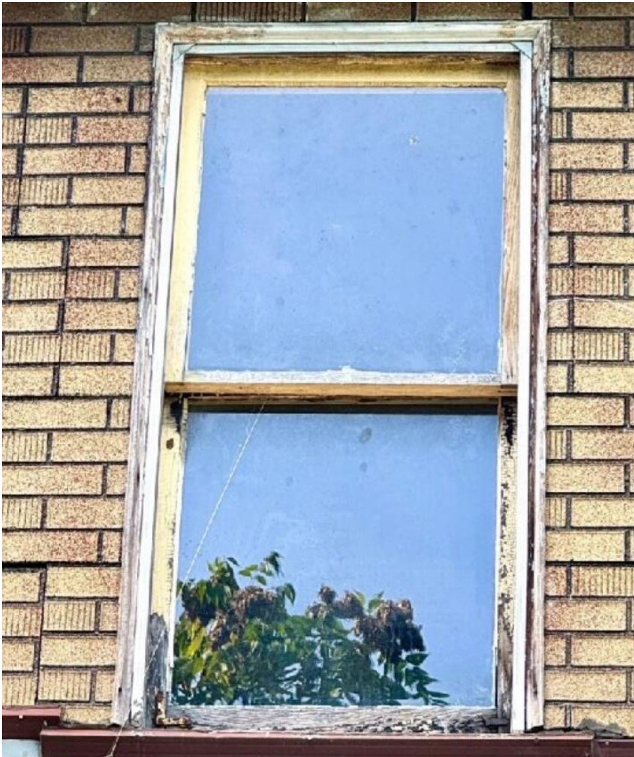
Window E- Photo by HDC staff, 10/3/2024
