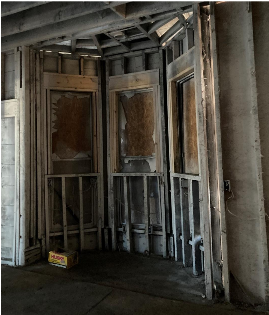
Interior, showing remaining historic east wall bay. Note that remnants from the windows which were damaged by the 2019 fire. Photo by HDC staff on 9/30/2024
