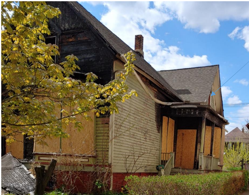
Conditions in 2019. Photo taken by Debra Walker, facing northwest.
