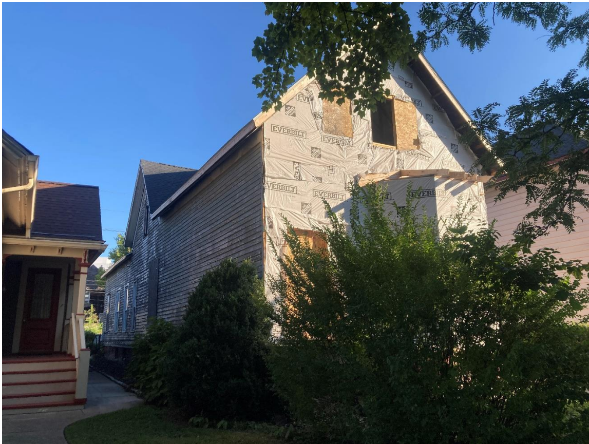
1628 Leverette, facing northeast. HDC staff photo taken 9/30/2024
