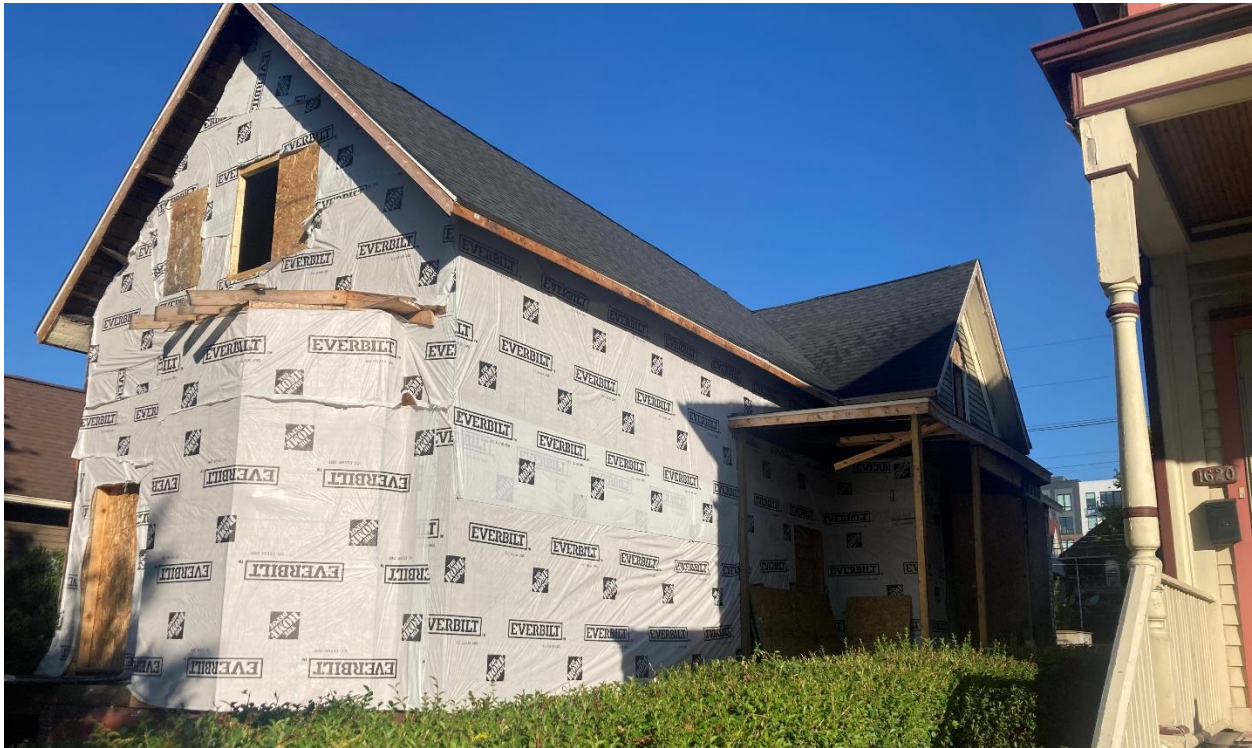
1628 Leverette, facing northeast. HDC staff photo taken 9/30/2024
