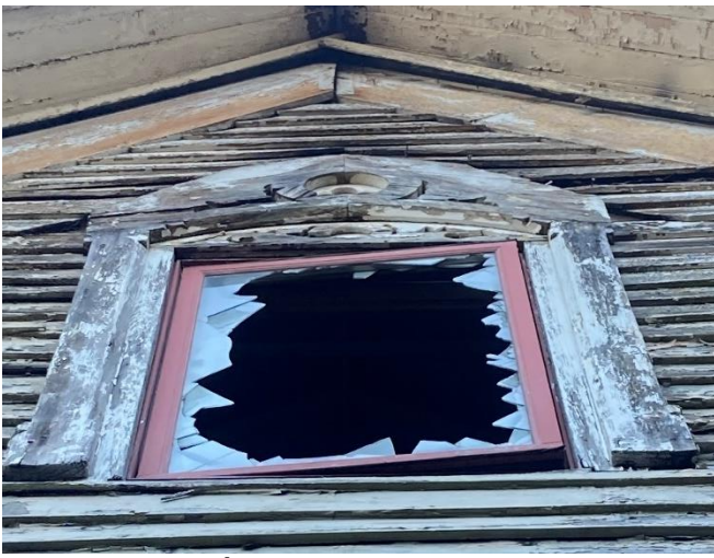
West side wall, 2 nd story gable end trim. Showing current conditions. 9/30/2024 by HDC staff. Note that the remaining damaged window is a non-historic vinyl casement
