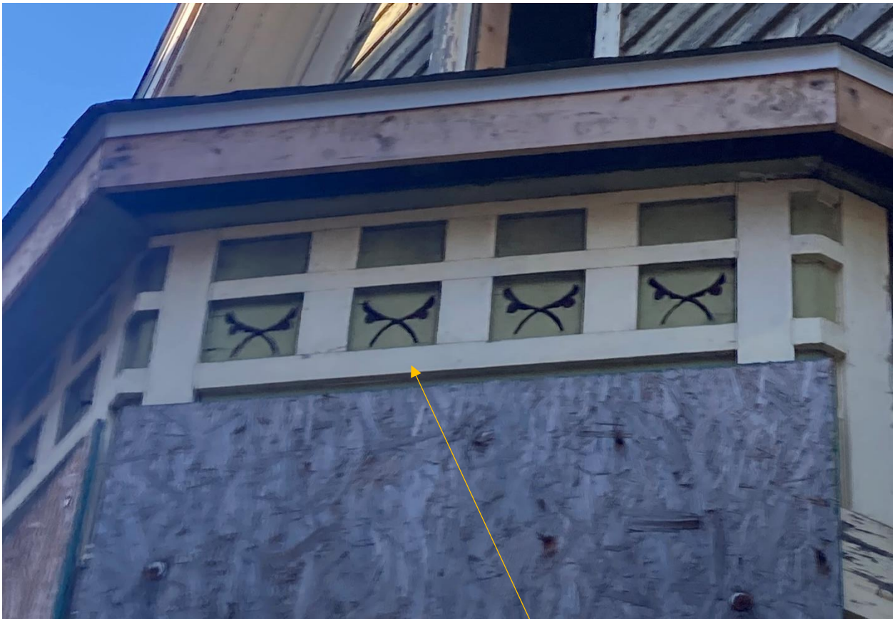
East wall bay, current conditions. Note that the historic wood detailing remains at this location despite the damage caused by the 2019 fire. Photo by HDC staff, 9/30/2024
