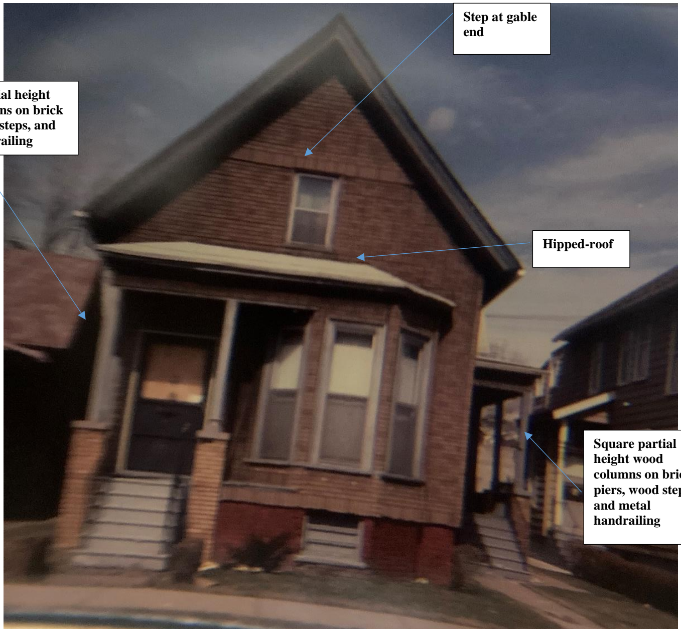
1628 Leverette, photo taken in 1983 by HDAB. Note that any exterior decorative detailing/trim is covered by the siding
