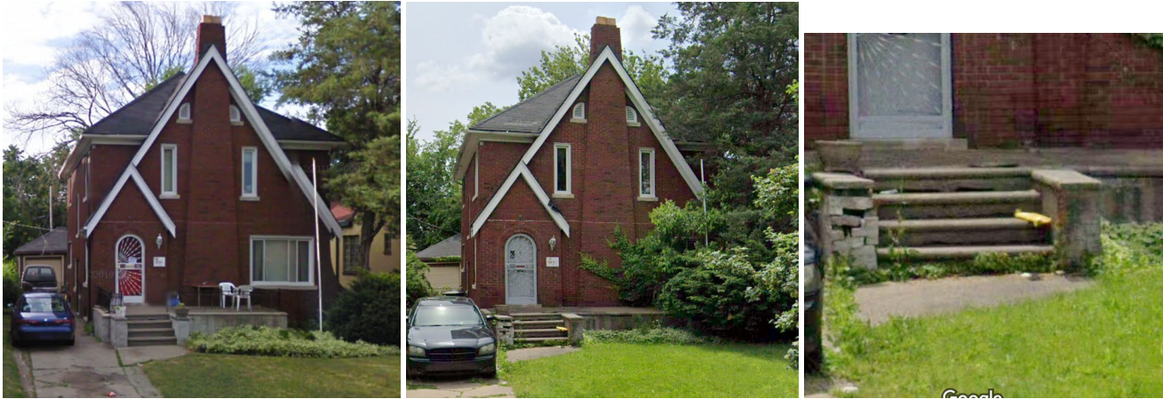
Google Street View images of 4881 Sturtevant. At left, 2009. Center, 2019. At right, zoomed into 2019 image showing brick decay.
