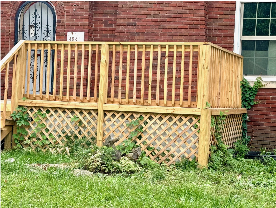
View of 4881 Sturtevant. It appears that part of the porch still exists below the deck. Staff photo, September 20, 2024.
