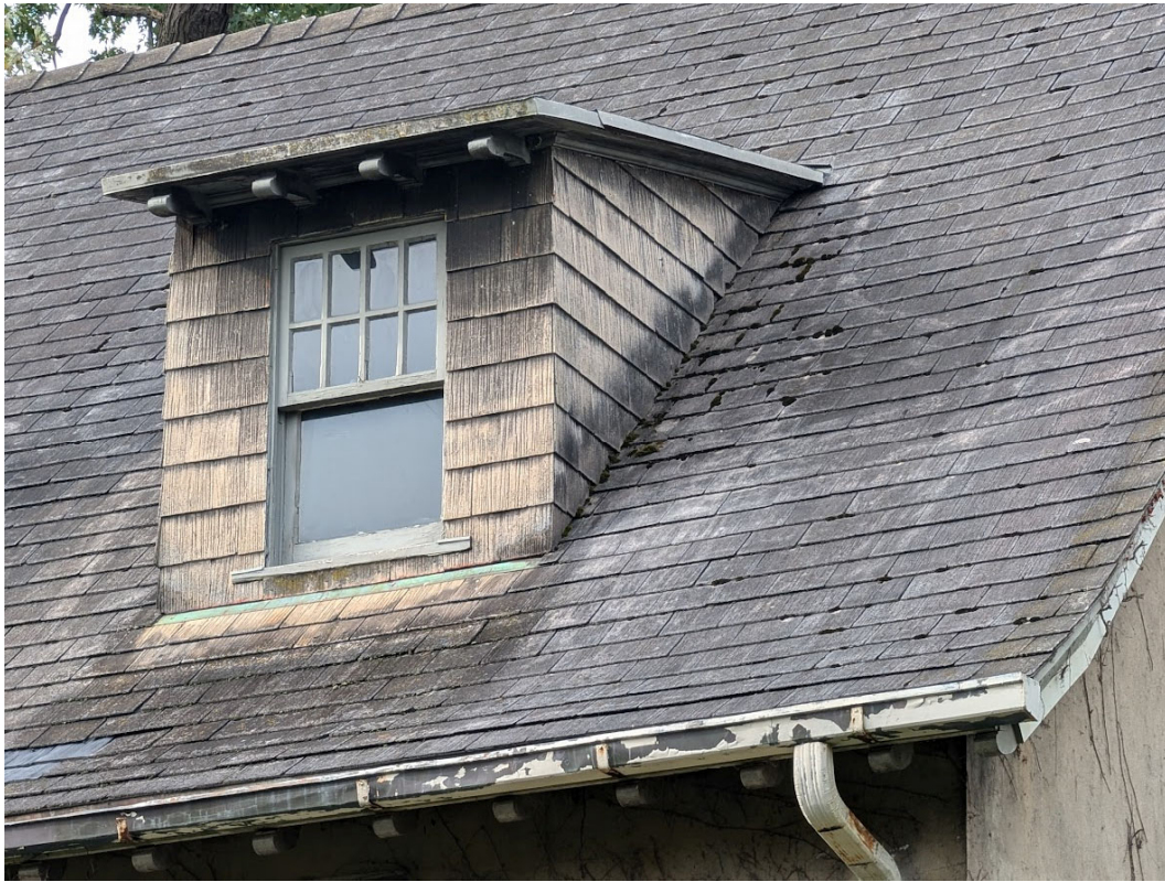
Detail view of roof conditions at northeast dormer. Staff photo, September 29, 2024.
