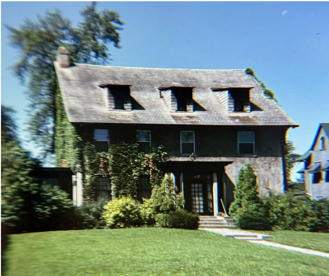
HDAB Designation photo, 1971
