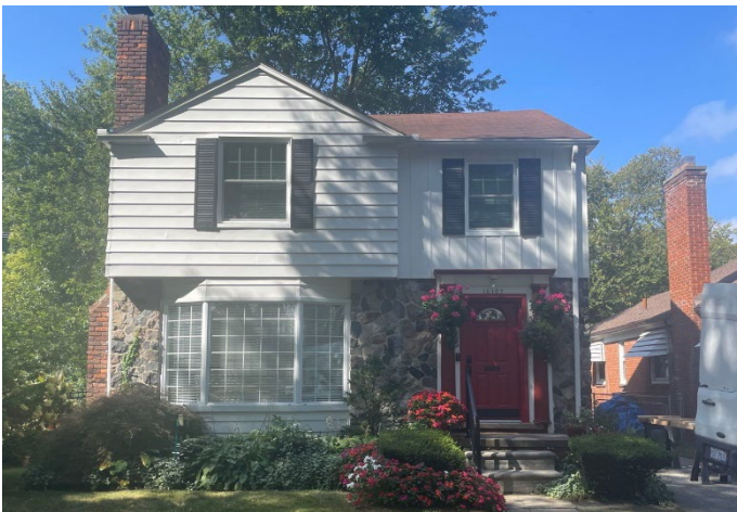
Site Photo 1, by Staff Sept. 19, 2024: (East) front elevation of house showing replaced windows and door.
