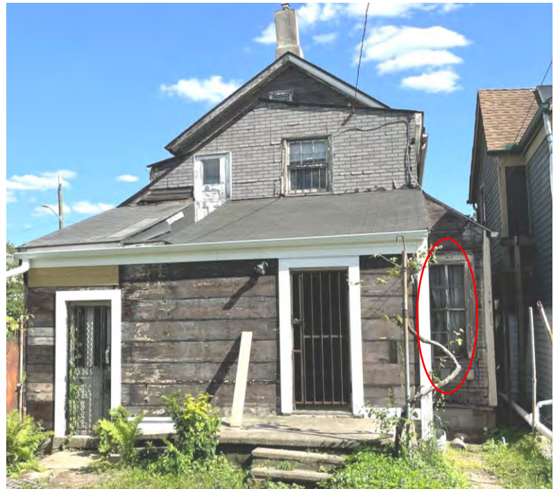
The outlines illustrate the approximate change to the rear wall for the sliding door, as well as the 10' x 13' wood deck with steps extending down on east and north sides. Door #7 is to be replaced with a half-panel/half-glass steel door.
