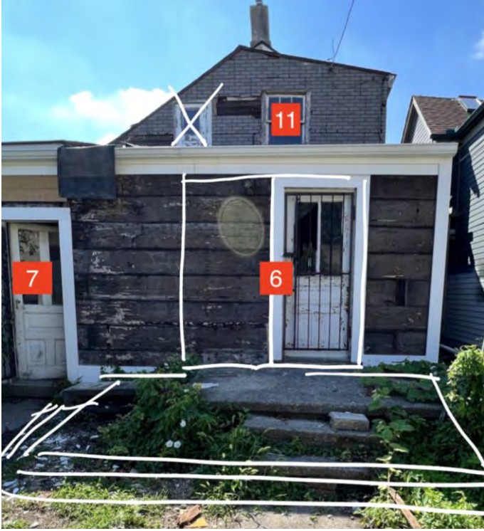
The outlines illustrate the approximate change to the rear wall for the sliding door, as well as the 10' x 13' wood deck with steps extending down on east and north sides. Door #7 is to be replaced with a half-panel/half-glass steel door.
