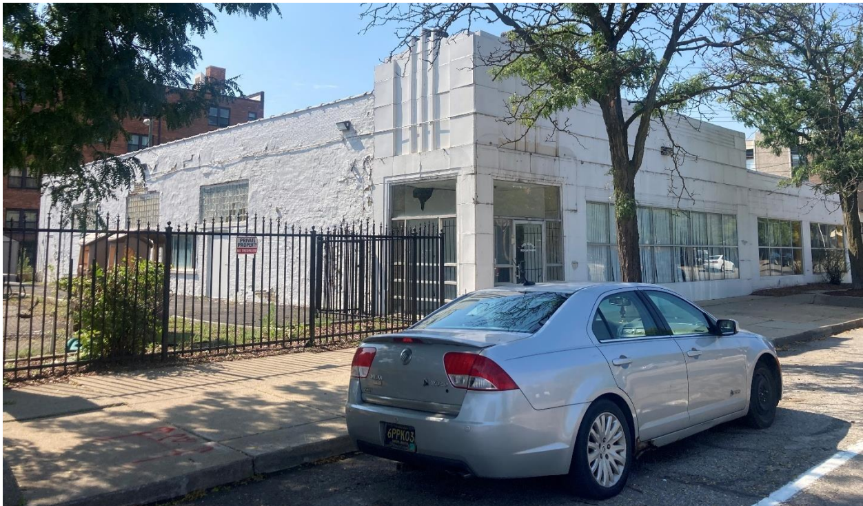
8007 Second Avenue, current conditions. Staff photo taken on 8/30/2024
