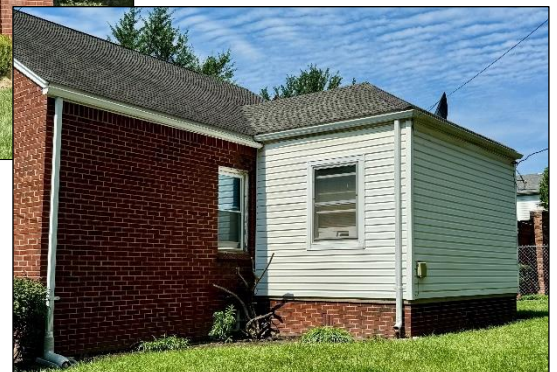
Rear wall and extension, Staff photo, August 27, 2024.
