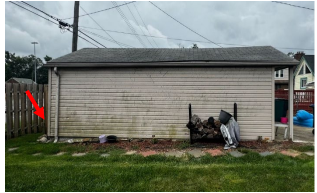
Site Photo 4, by Applicant, showing north side of the existing garage. The arrow indicates the location of past vehicle impact.
