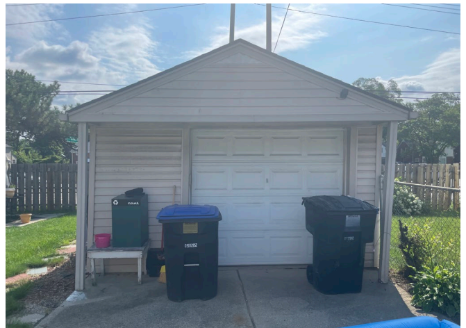
Site Photo 2, by Staff July 25, 2024: (West) front elevation of the existing garage.
