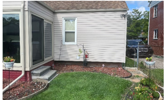
Site Photo 5, by Staff, July 25, 2024, showing location of proposed concrete patio.
