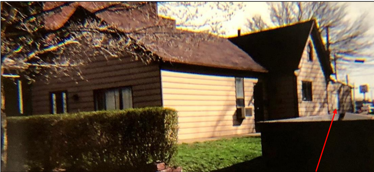
1984 designation photo – view from Wabash showing front and south-side elevations, HDAB. The pre-1921 rear addition, which had a shed roof, is partially visible in this photo (red arrow).
