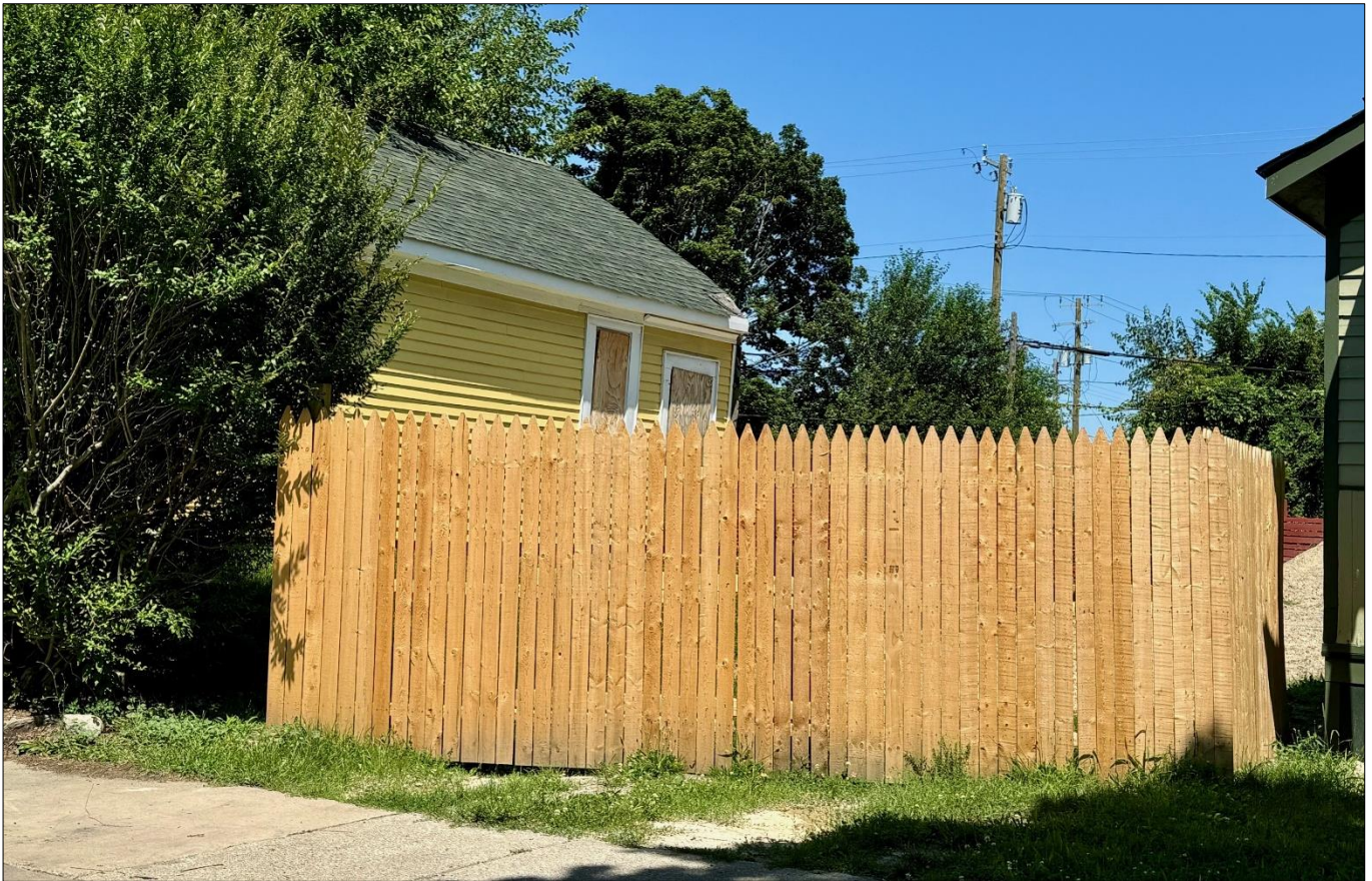
Current view from Wabash sidewalk looking northeast toward alley. Staff photo, July 26, 2024. The stockade fence was erected without HDC approval. Applicant states it was installed temporarily to enclose the lot which has an excavated and open foundation wall at the rear of the structure.
