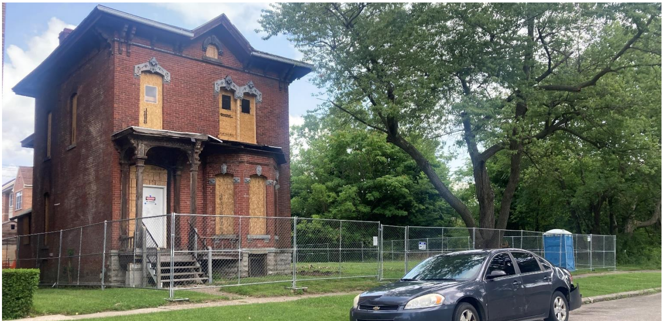
3628-3644 Lincoln, facing southeast. Current conditions. Vacant lot extends to the right in this image. Staff photo taken on 7/29/2024
