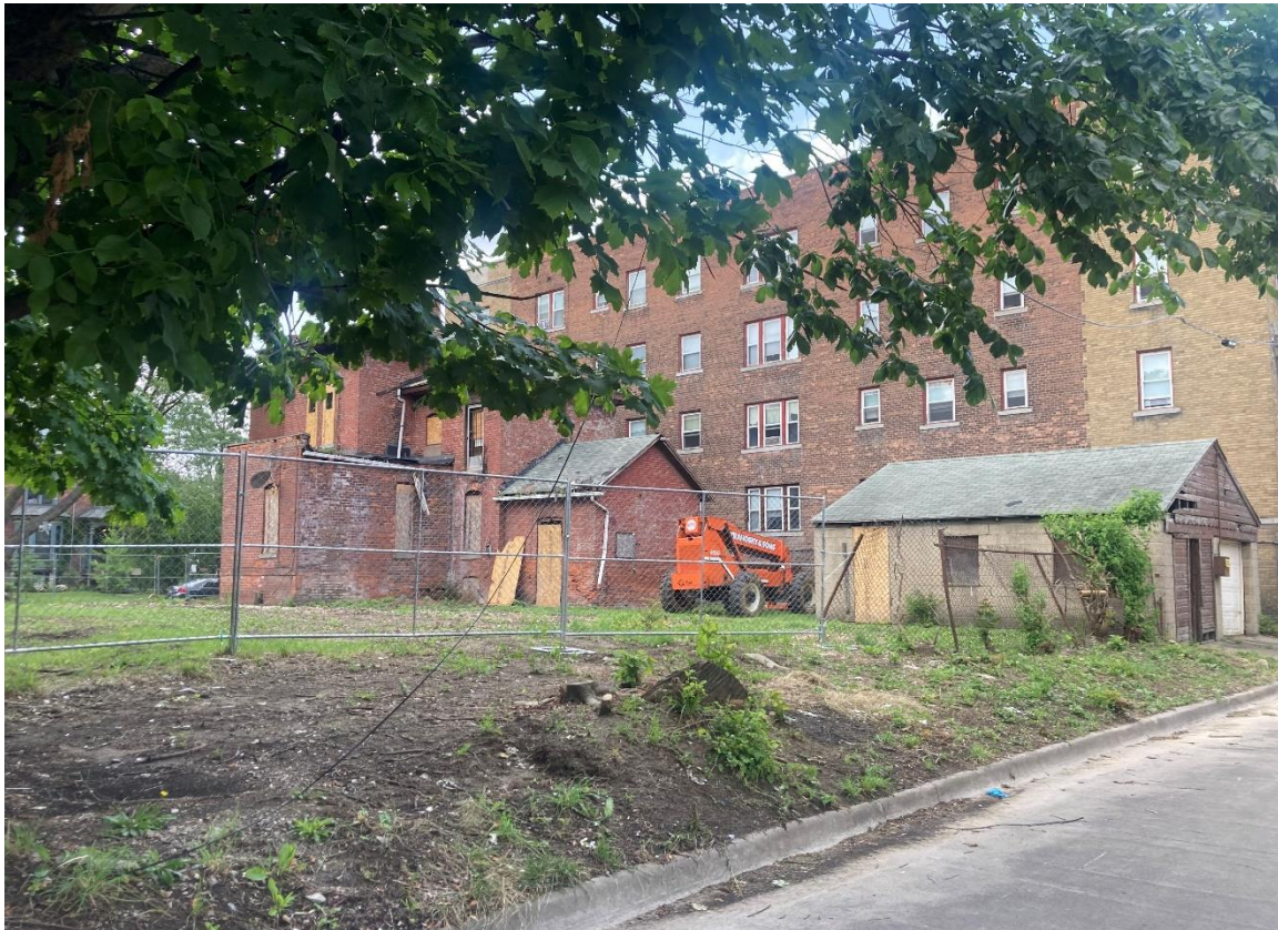
3628-3644 Lincoln, facing northwest toward rear of lots. Current conditions. Staff photo taken on 7/29/2024
