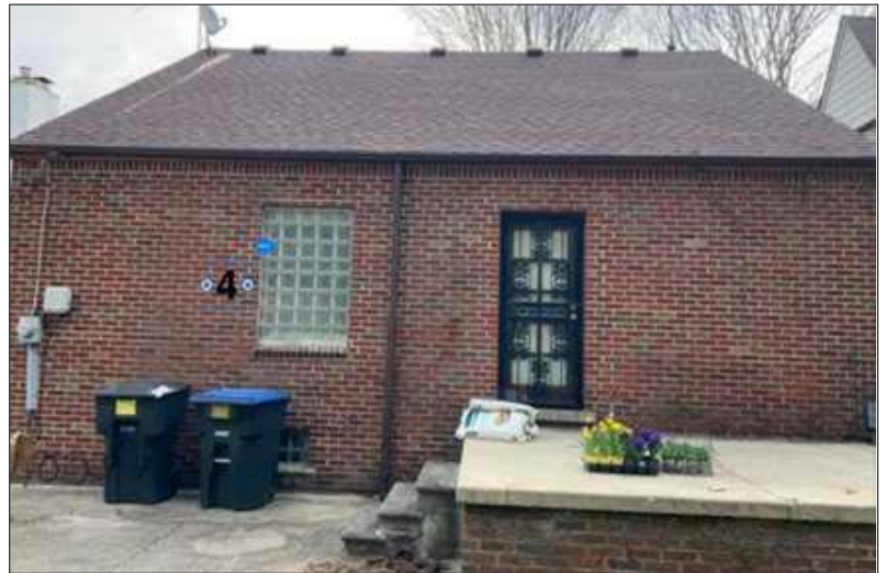
Applicant photo of rear wall with third glass block opening.
