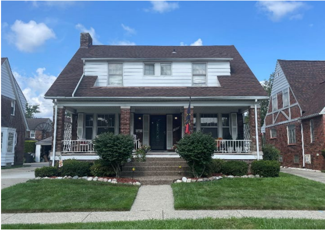
Site Photo 1, by Staff July 25, 2024: (East) front elevation showing original wood windows.
