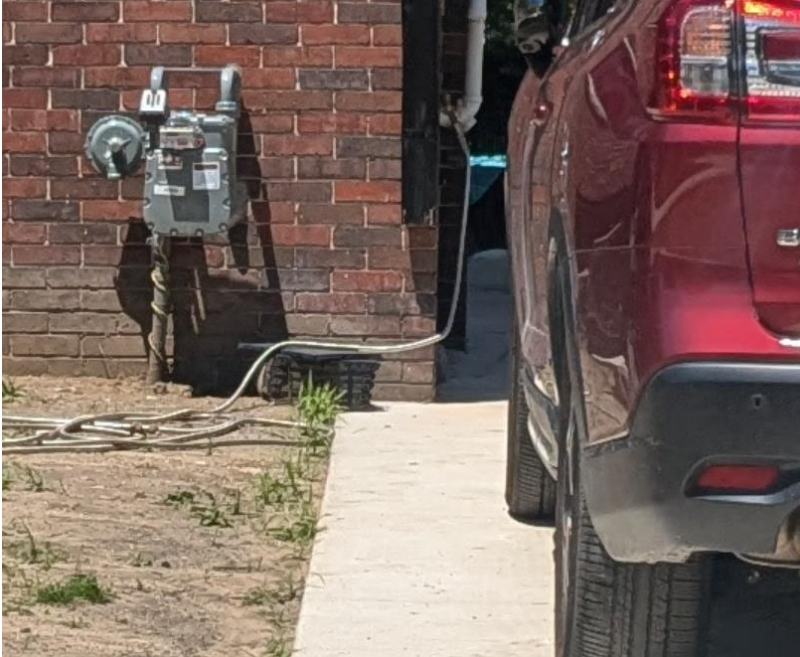
July 2024 staff photo showing inappropriate overlap of driveway with front façade of the house.
