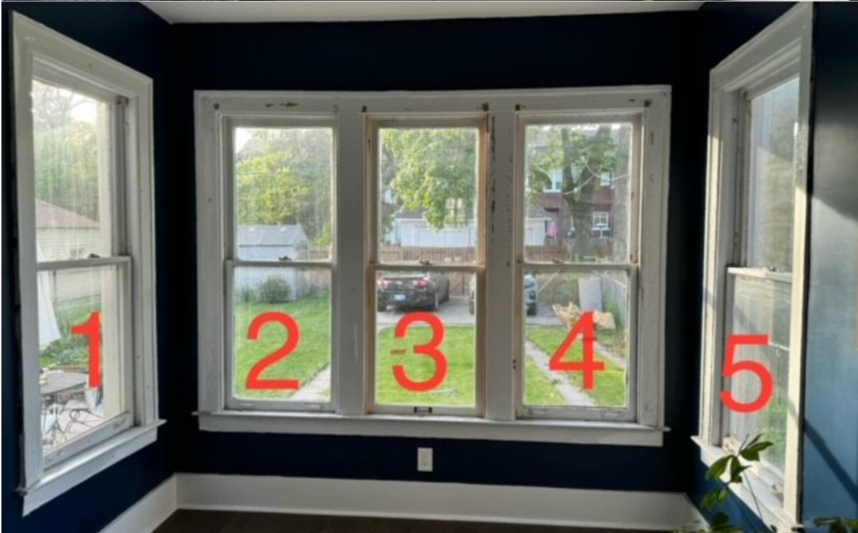
Above: Second-floor windows; below: first-floor windows. Photos from application materials.
