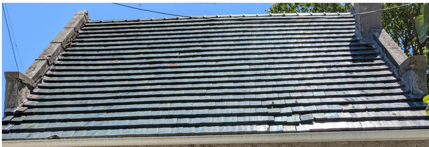
North (alley-facing) plane of the roof. July 2024 photo by staff.
