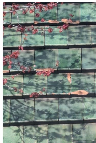
Application photos showing damaged areas of roofing. Please see application materials for additional photos.
