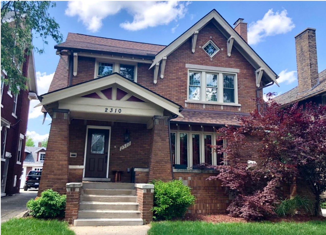
Façade, east-facing wall. Staff photo, May 22, 2024.
