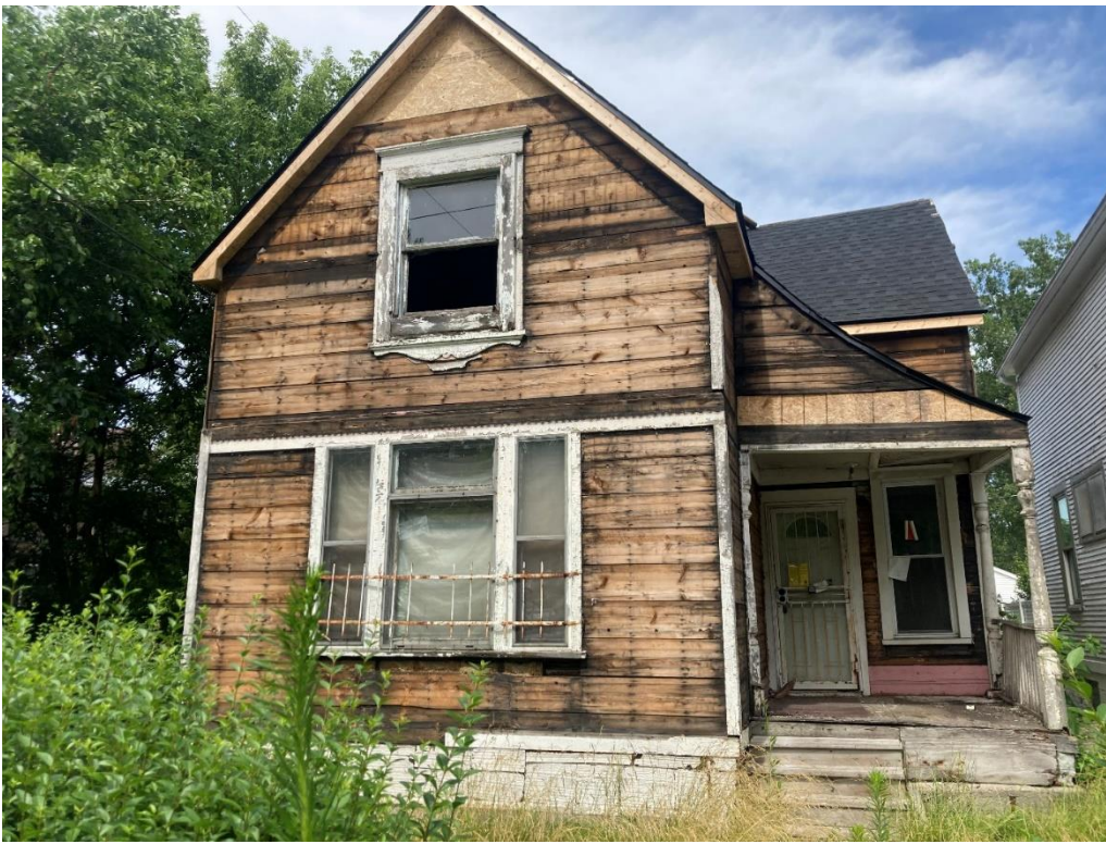
1480 Shipherd, front façade. Current condition. Staff photo taken on 6/25/2024. Note that only small areas of corner board trim, the windows; and porch posts, pilasters, floor, steps, and railing remain at the front façade. All other siding and detailing at the walls and roof have been removed without HDC approval.
