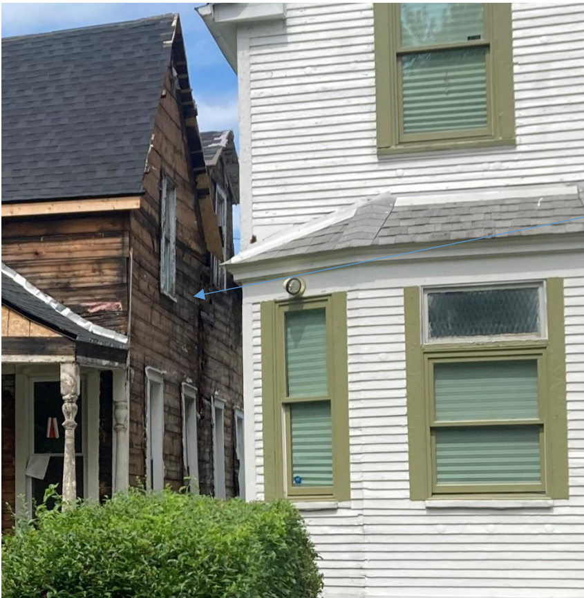
1480 Shipherd, front façade. Current condition. Staff photo taken on 6/25/2024. Note that only small areas of corner board trim, the windows; and porch posts, pilasters, floor, steps, and railing remain at the front façade. All other siding and detailing at the walls and roof have been removed without HDC approval.
