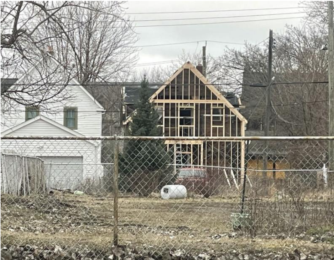
1480 Shipherd, rear addition. Photo taken by HDC staff on 2/28/2024
