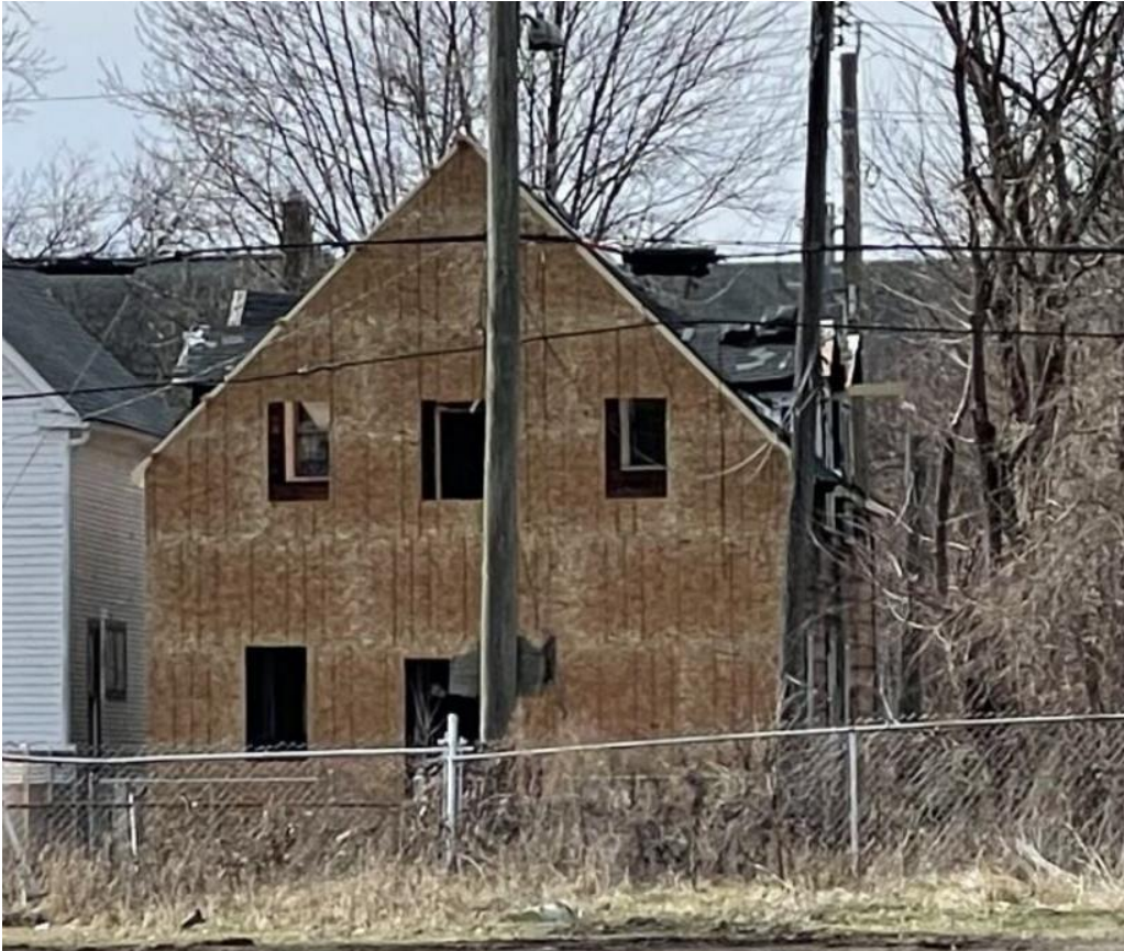
1480 Shipherd, rear addition. Photo taken by HDC staff on 3/1/2024
