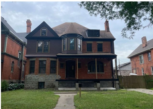
Site Photo 1, by Staff June 26, 2024: (North) front elevation showing current conditions.
