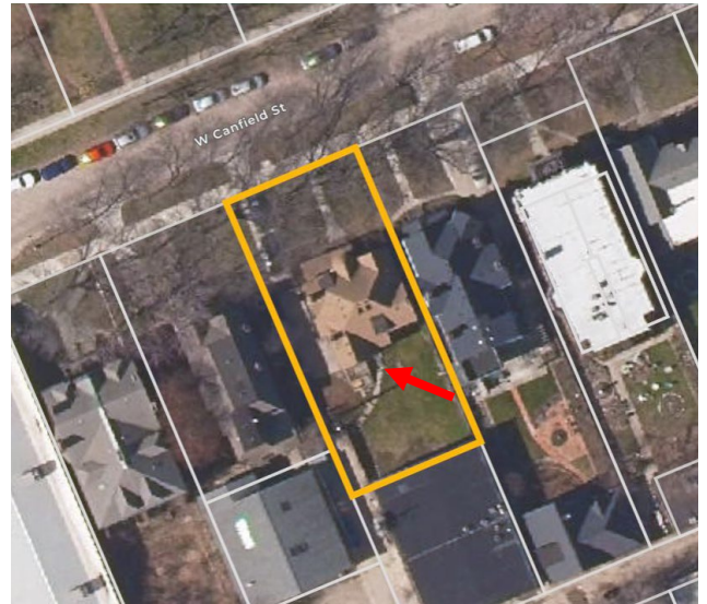
Aerial 1 of Parcel # 04000899, by Detroit Parcel Viewer, showing the location of proposed basement entrance structure (arrow).
