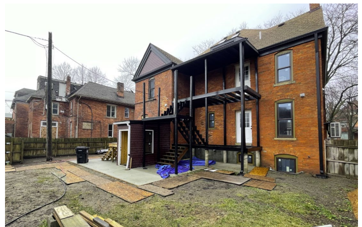
Site Photo 2, by Applicant June 2024: (South) rear elevation showing current conditions.
