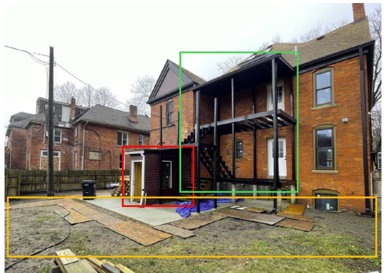
Site Photo 4, by Applicant, June 2024: (South) rear elevation location showing locations of work: red and gold boxed areas are included in this proposal, the green box is for a future application.
