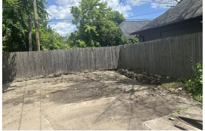
Site Photo 3, by Applicant: (facing southeast) rear southeast corner of the property showing location for the proposed garage.
