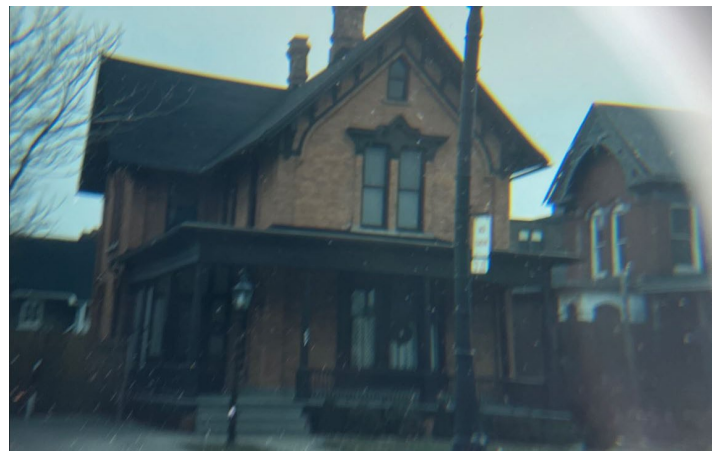
Image HDC hard files, 1973: (North) front elevation showing original windows.
