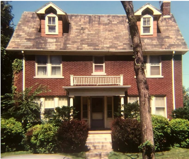
1978 photo by the Historic Designation Advisory Board. Note balustrade and slate roof that no longer remain.
