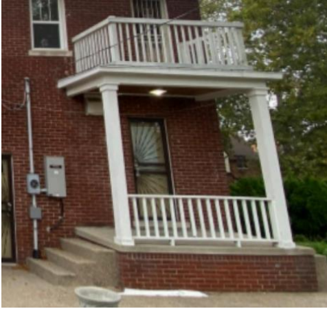
Historic rear (east) porch. Photo from application materials.
