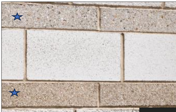
Left: Photo from Echelon Masonry’s Facebook page. Rows of Trendstone Plus units are identified with blue stars. This example shows the product in a size different than proposed by the applicant and is very likely “44F” (shown below). It is used as an alternating course with traditionally sized CMU.
