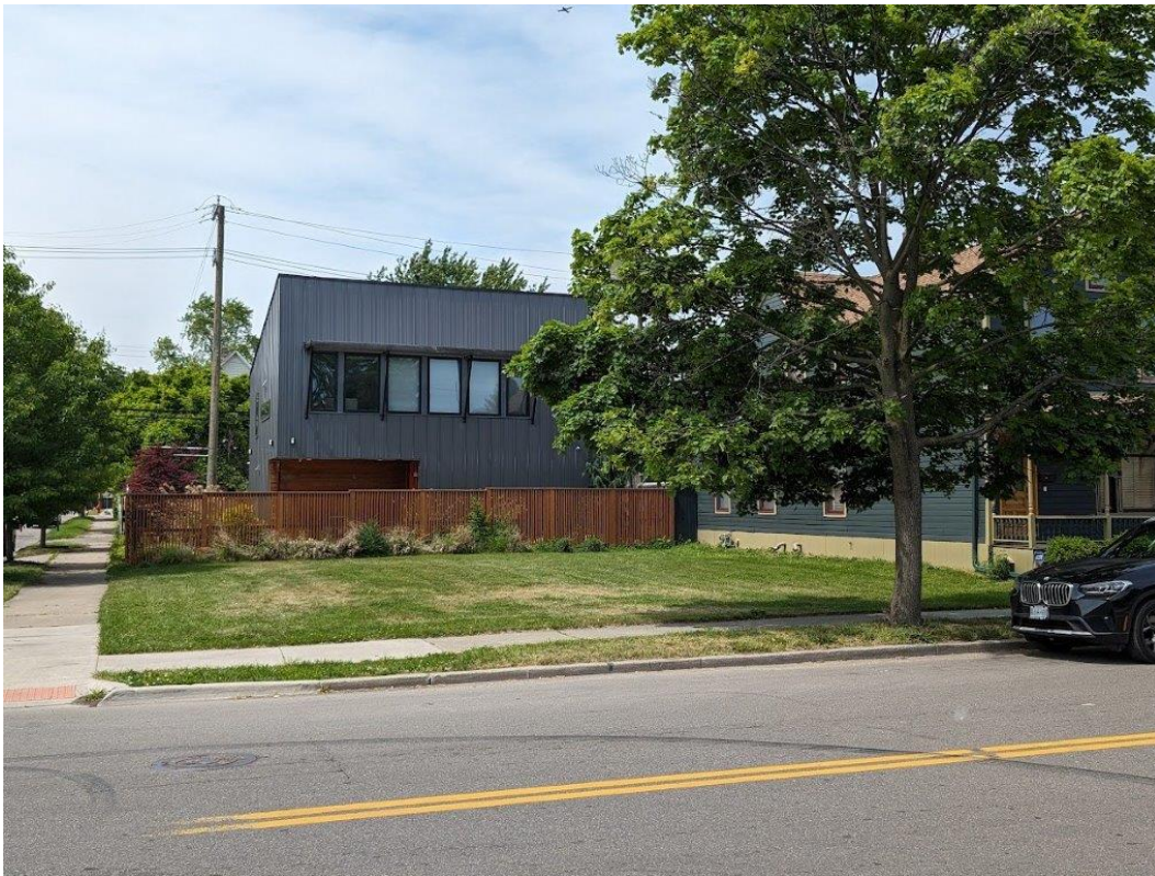
View of existing conditions at 1566 Bagley, view to the north from Bagley. Staff photo, March 24, 2024.
