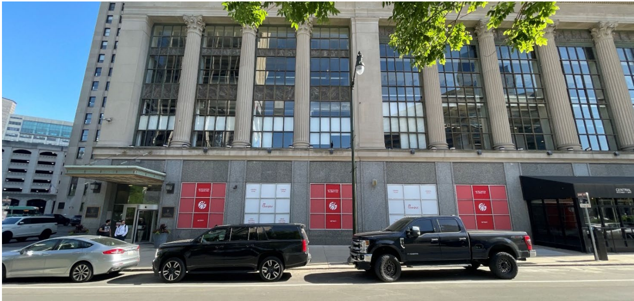
Site Photo 1, by Staff May 22, 2024: (facing north) showing existing storefront at northeast corner of the building, facing Cadillac Square.
