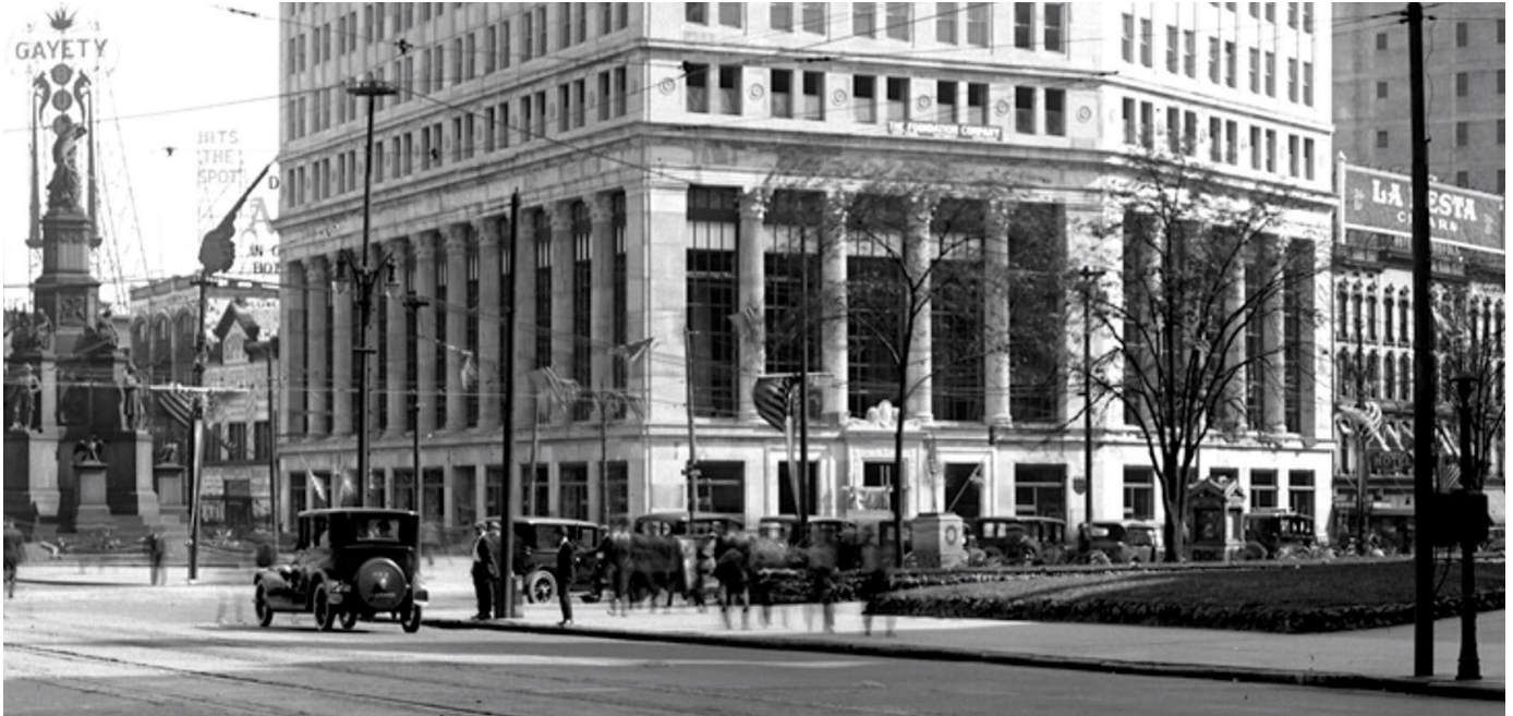
Figure 1, by Burton Collection, date unknown: (facing southeast) showing corner storefront at northwest corner of Woodward and Cadillac Square, showing original limestone façade surrounding the storefront and main entrance.
