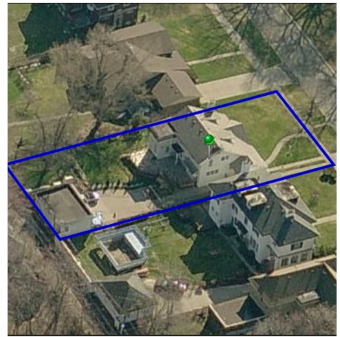
Aerial 2 of Parcel # 03002670. by Eagleview.com, showing 2006 view of rear elevation with new deck and original rear porch roof and post still in place.
