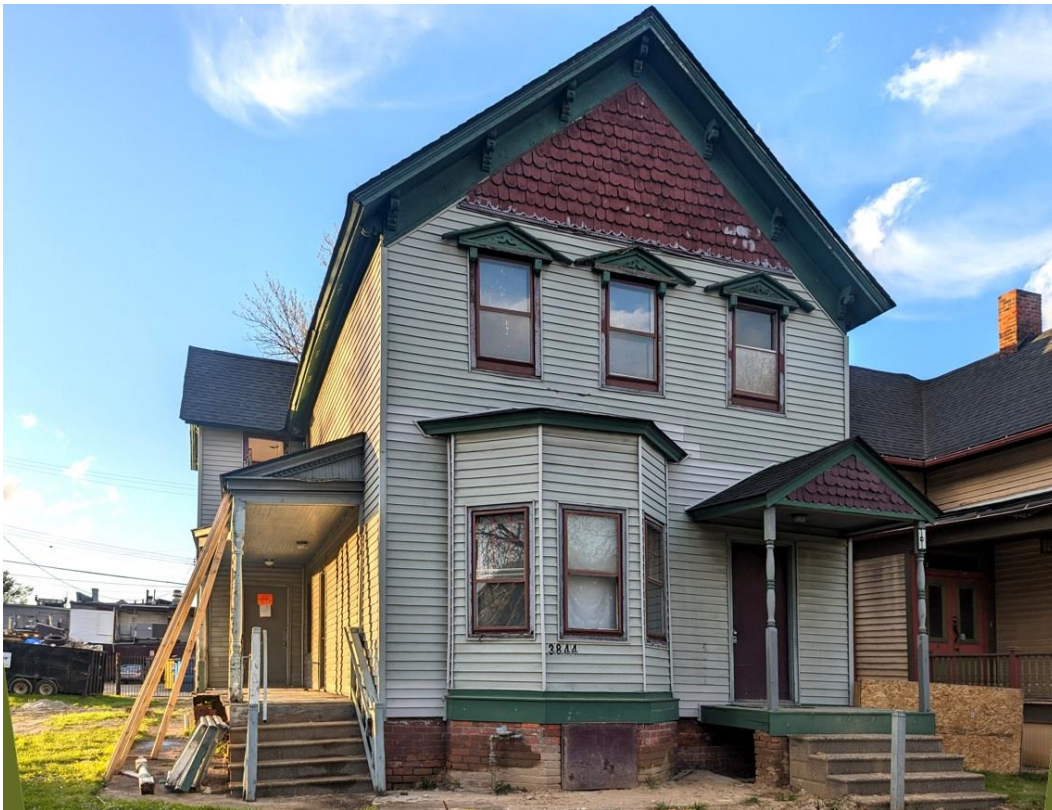
April 2024 photo by staff. Note porch elements removed without approval are sitting on the ground at the lower left corner of this image.
